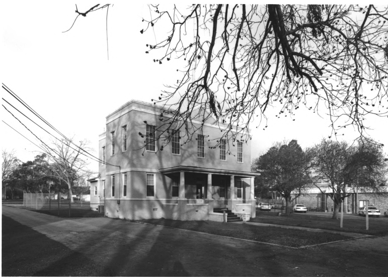
CANDLER COUNTY JAIL METTER, CANDLER COUNTY, GEORGIA PHOTOGRAPH 14 OF 14
