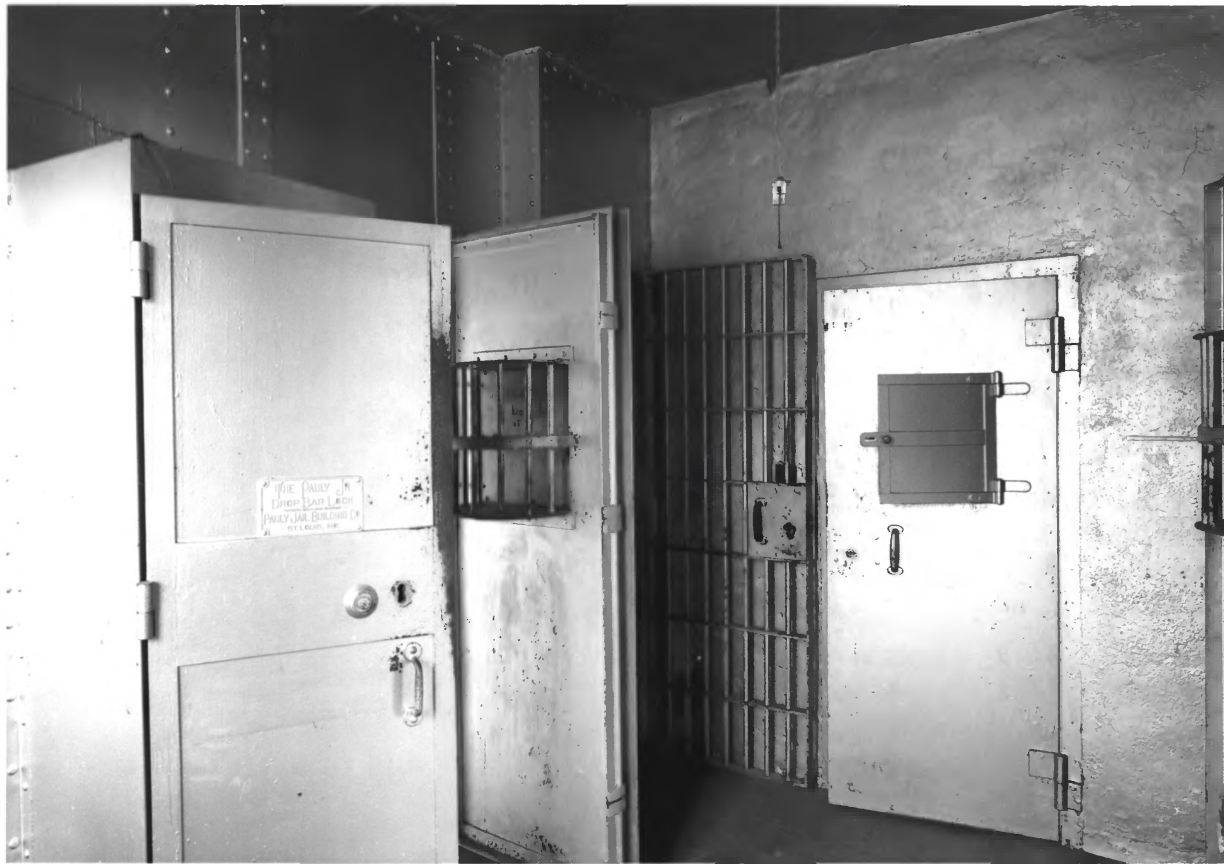
CANDLER COUNTY JAIL METTER, CANDLER COUNTY, GEORGIA PHOTOGRAPH 10 OF 14
