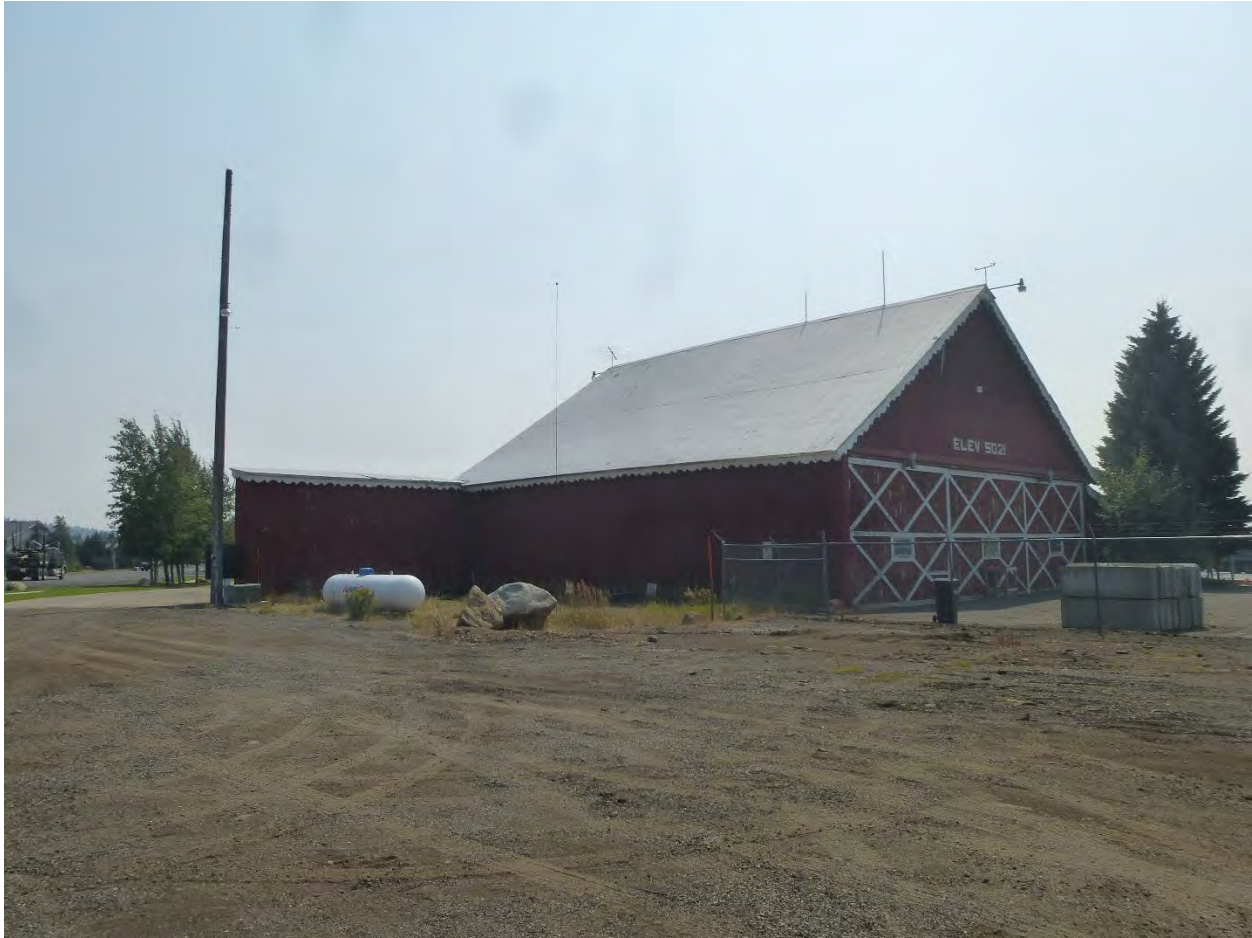
Photo #8: (ID_Valley County_Johnson Flying Service Hangar_0008) Northeast and northwest elevations, camera facing south.
