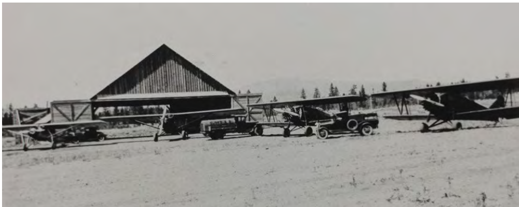
Figure 5. Johnson Flying Service Hangar, circa 1935, showing original hangar doors. Photo courtesy of Mike Dorris.
