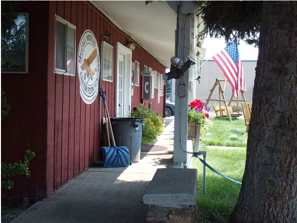
Photo # 12 (ID_Valley County_Johnson Flying Service Hangar_0012) Southwest elevation, camera facing southeast.
