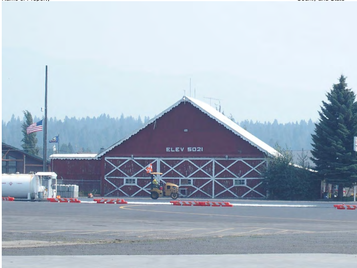
Photo #2. (ID_Valley County_Johnson Flying Service Hangar_000) Northwest elevation, camera facing southeast.
