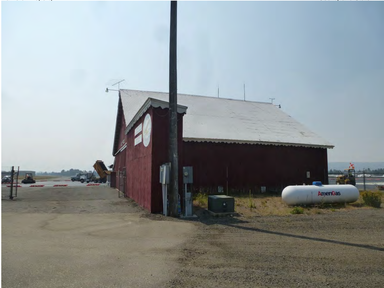
Photo #6: (ID_Valley County_Johnson Flying Service Hangar_0006) Southeast and northeast elevations, camera facing northwest showing hangar storage compartment.
