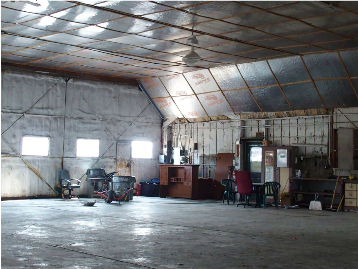
Photo # 13: (ID_Valley County_Johnson Flying Service Hangar_0013) Interior view, camera facing northeast.
