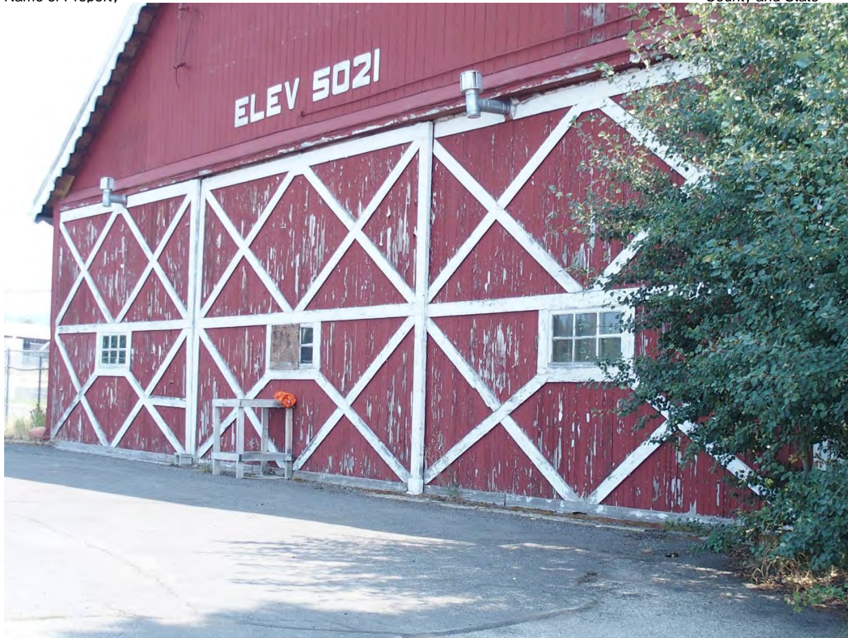
Photo #9 (ID_Valley County_Johnson Flying Service Hangar_0009) Northwest elevation, camera facing southeast.
