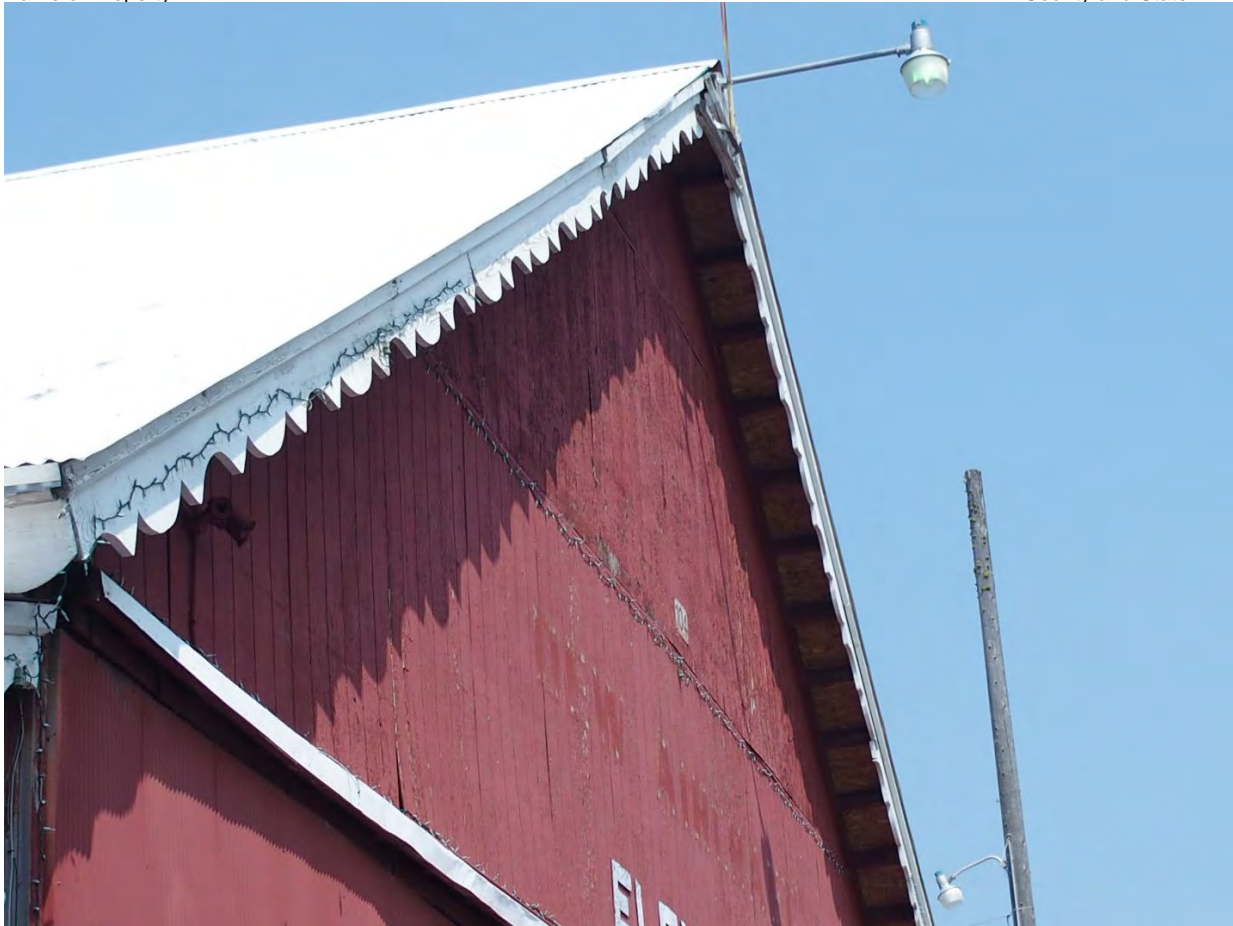
Photo # 11 (ID_Valley County_Johnson Flying Service Hangar_0011) Southeast elevation, detail of trim.
