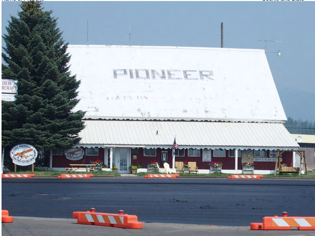
Photo #3 (ID_Valley County_Johnson Flying Service Hangar_0003) Façade, southwest elevation, camera facing northeast.
