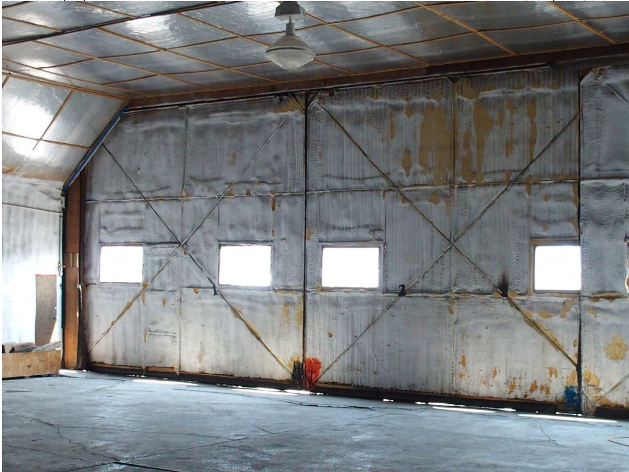
Photo # 14: (ID_Valley County_Johnson Flying Service Hangar_0014) Interior view, camera facing northwest.
