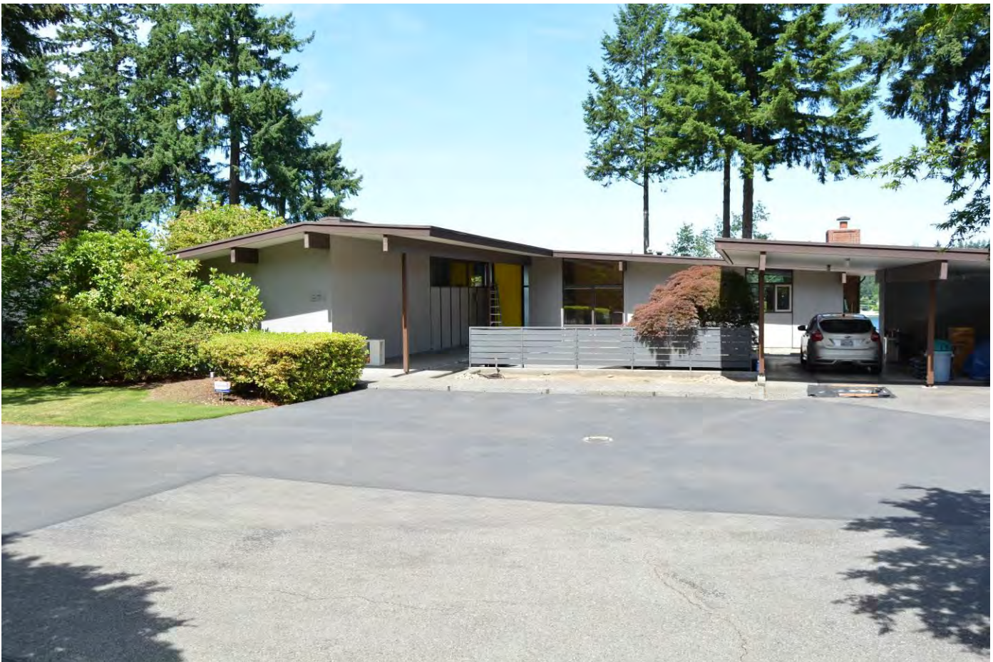
1 of 25. Main/West façade showing entry courtyard and carport.
