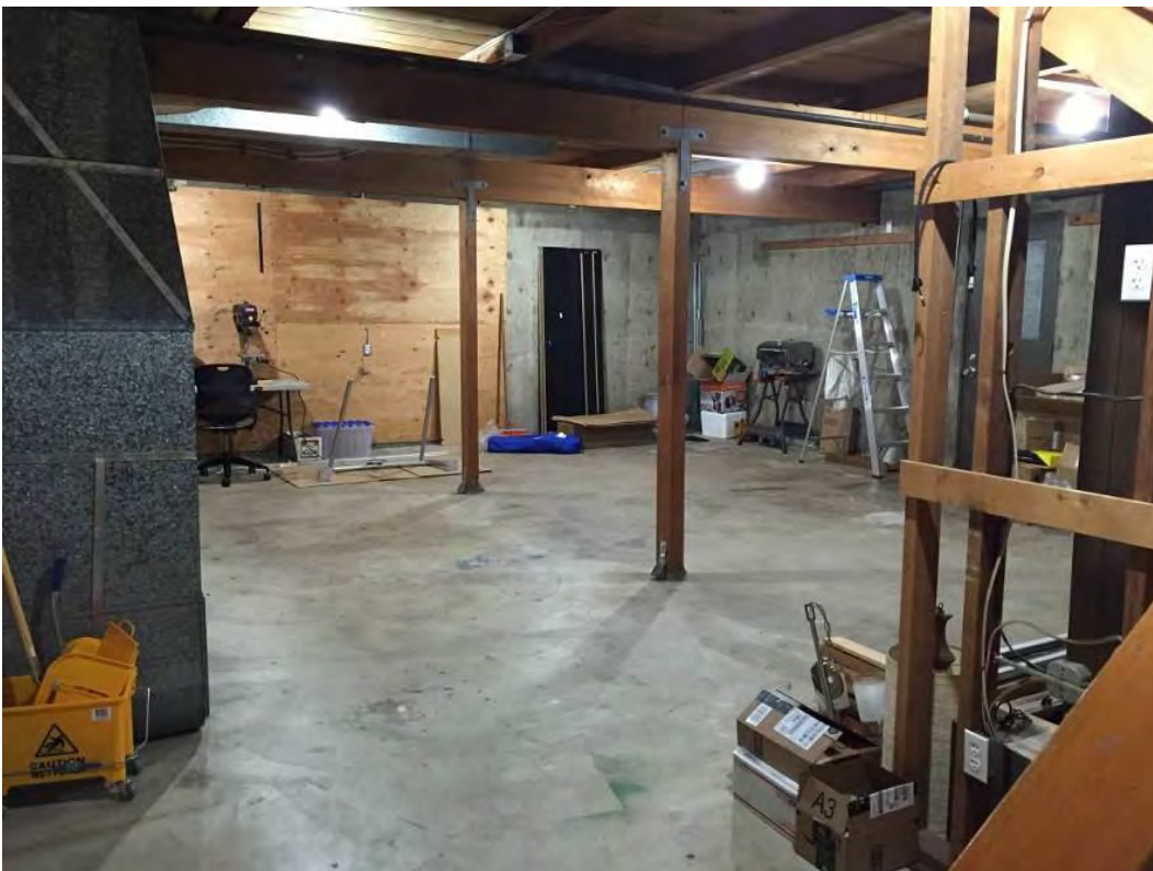
24 of 25. Unfinished partial basement.
