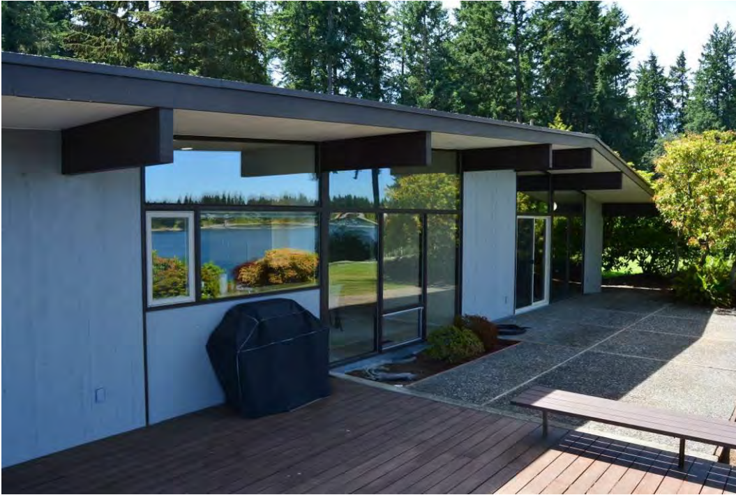
6 of 25. Rear/East facade.
