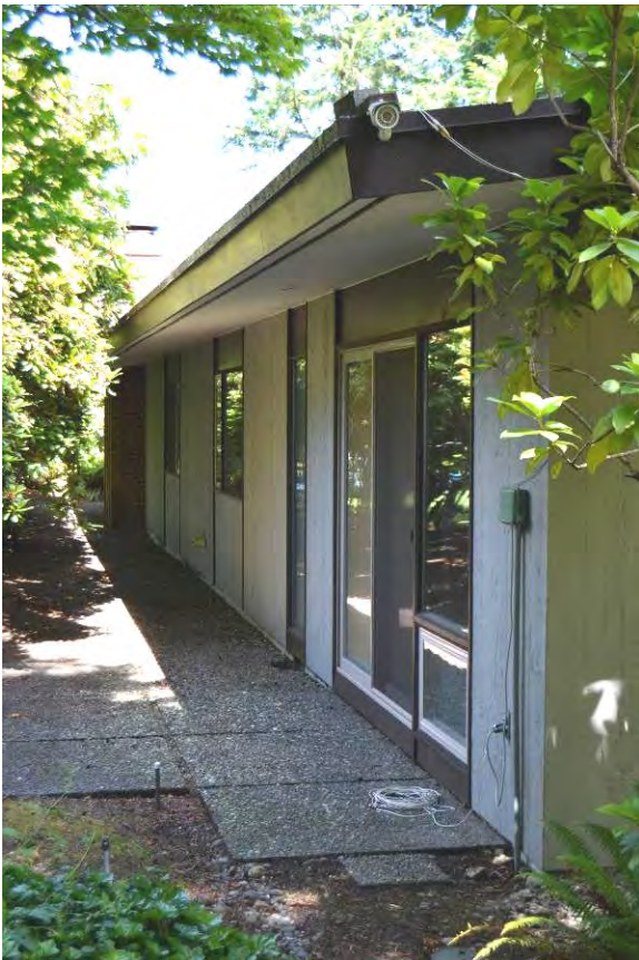
5 of 25. North façade showing master bedroom patio.
