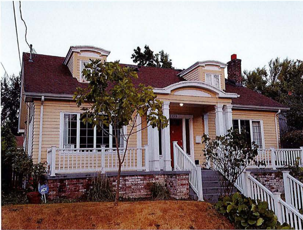
34 of 37 – House at 2806 31 st Avenue S.
