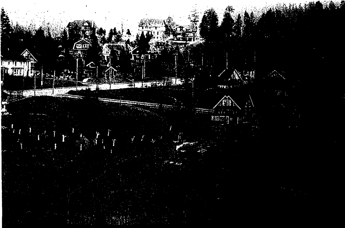
View north towards S McClellan Street and 32nd Avenue S. Street interchange. Courtesy of Rainier Valley Historical Society.
