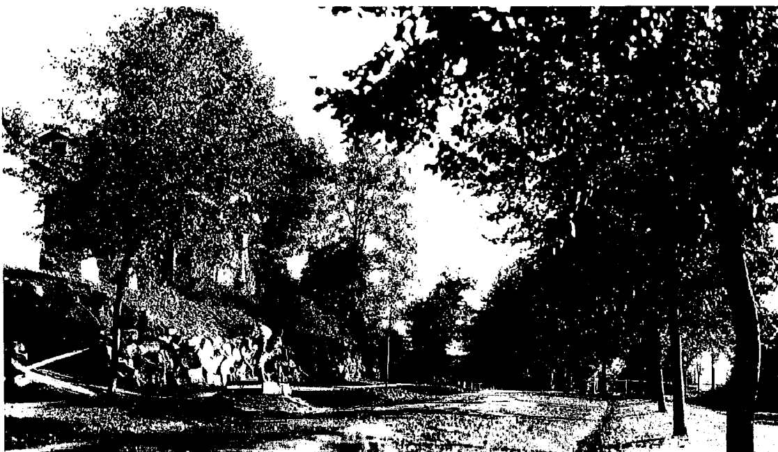
Mount Baker Drive, 1924. Courtesy Seattle Municipal Archives, Engineering Department Photographic Negatives, Record Series 2613-07, Item no. 57521.
