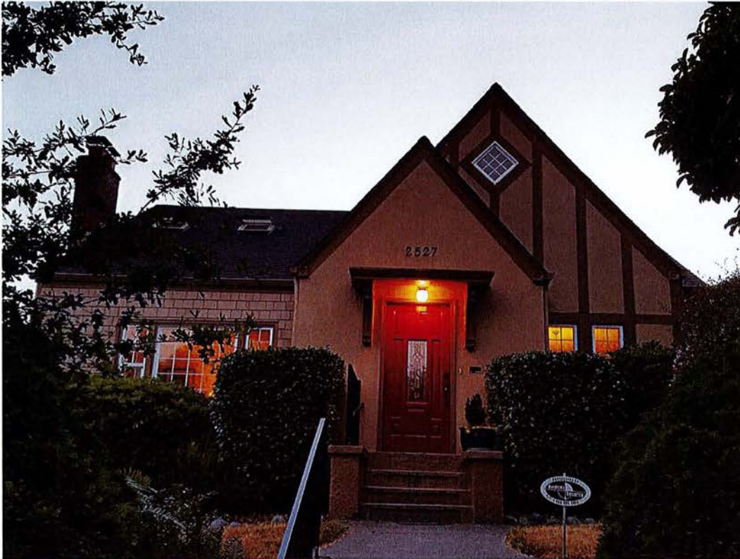
32 of 37 – House at 2527 31 st Avenue S.
