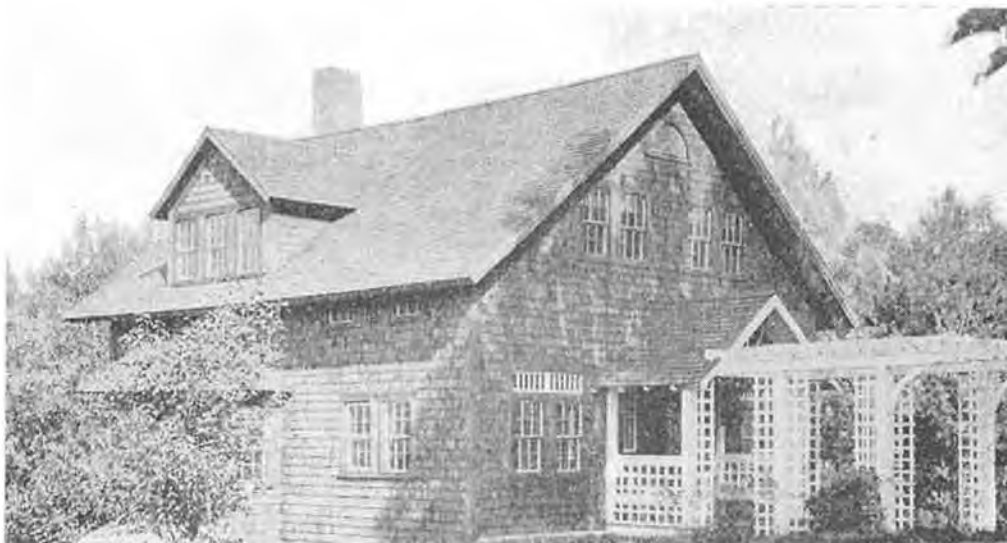
HP 7: The Lodge (#3), photographed in 1919 and showing alterations of previous year.
