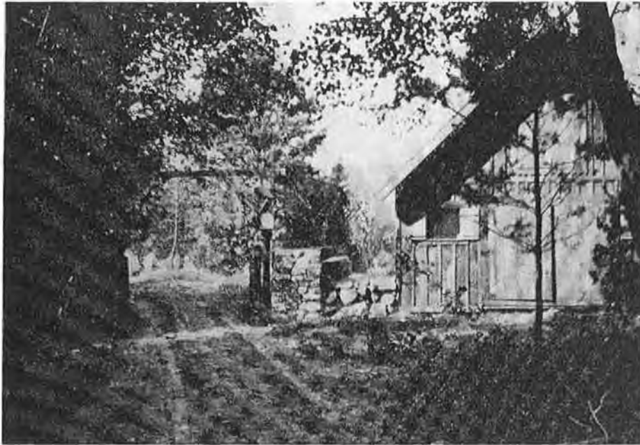
HP 11: Main road into camp, showing gate posts (#39) and Craft Shop (#6).
