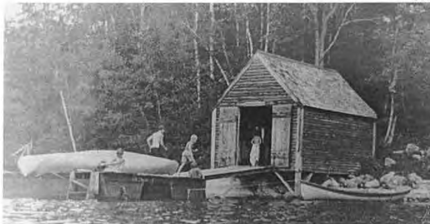
HP 36: Waingunga (#29), photographed 1905 shortly after its relocation to this spot at camp.
