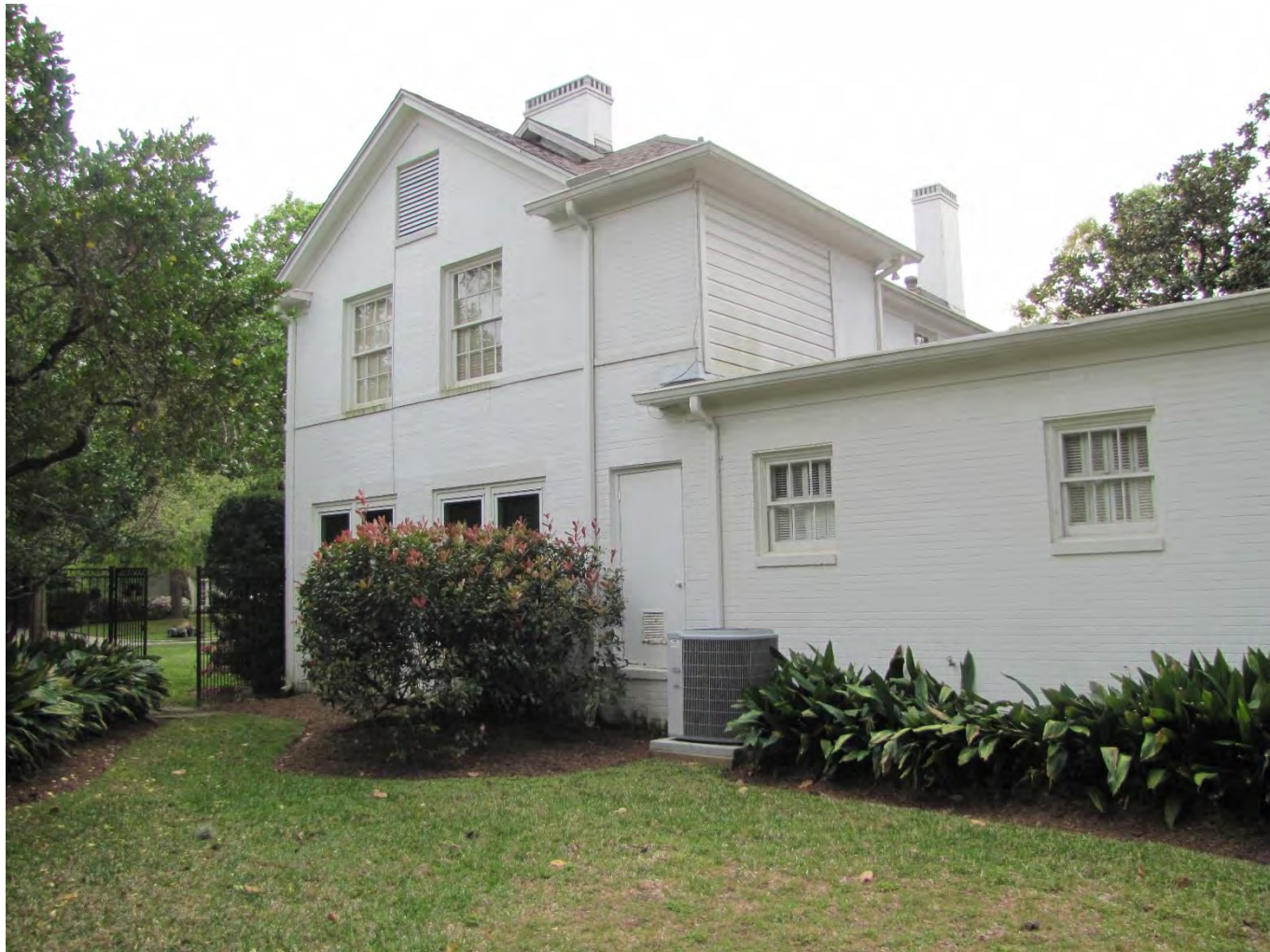
Photo 13: East elevation of east wing and 1970 addition. Camera facing west.
