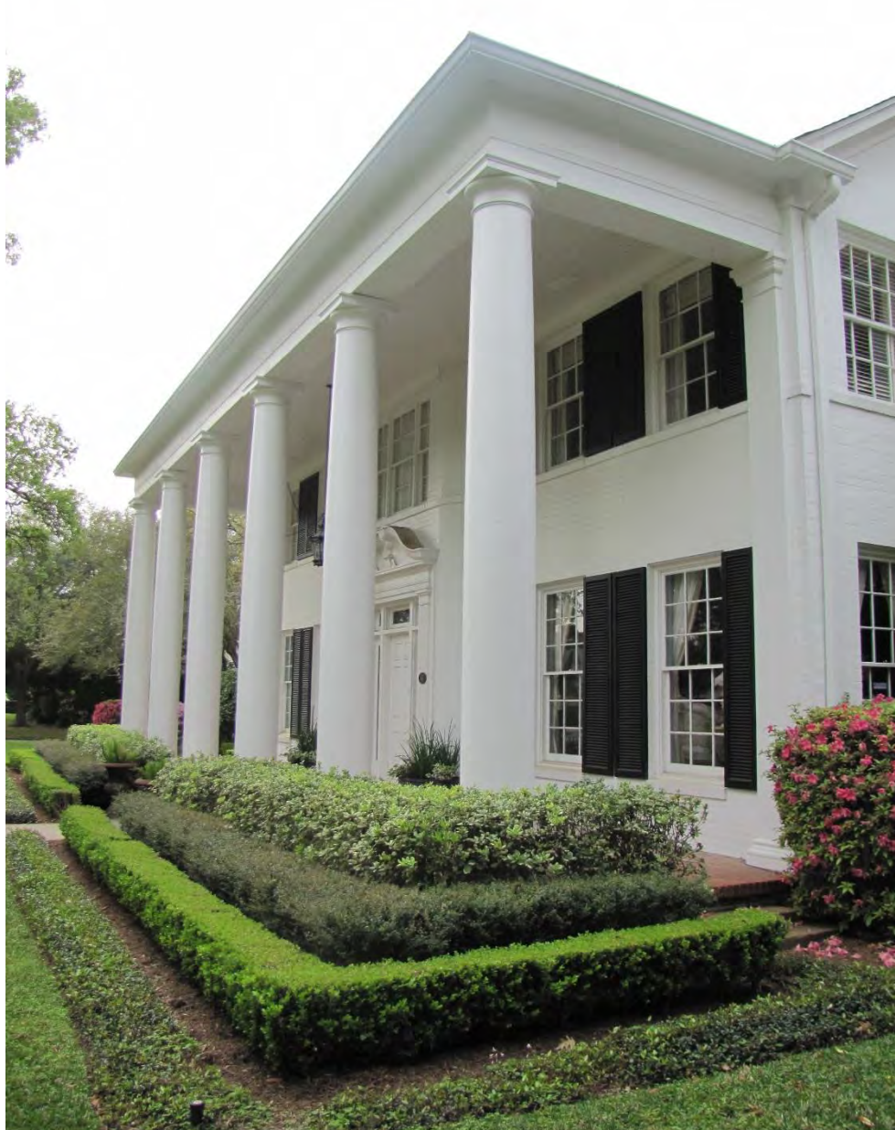
Photo 5: View of portico and landscaped vegetation. Camera facing northwest.
