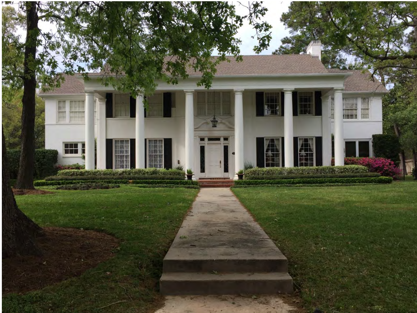
Photo 1: Primary (south) elevation showing two-story main block with recessed wings. Camera facing north.
