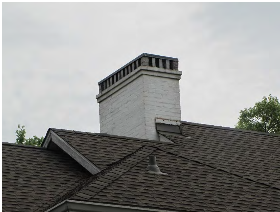
Photo 16: View of east chimney. Camera facing south.
