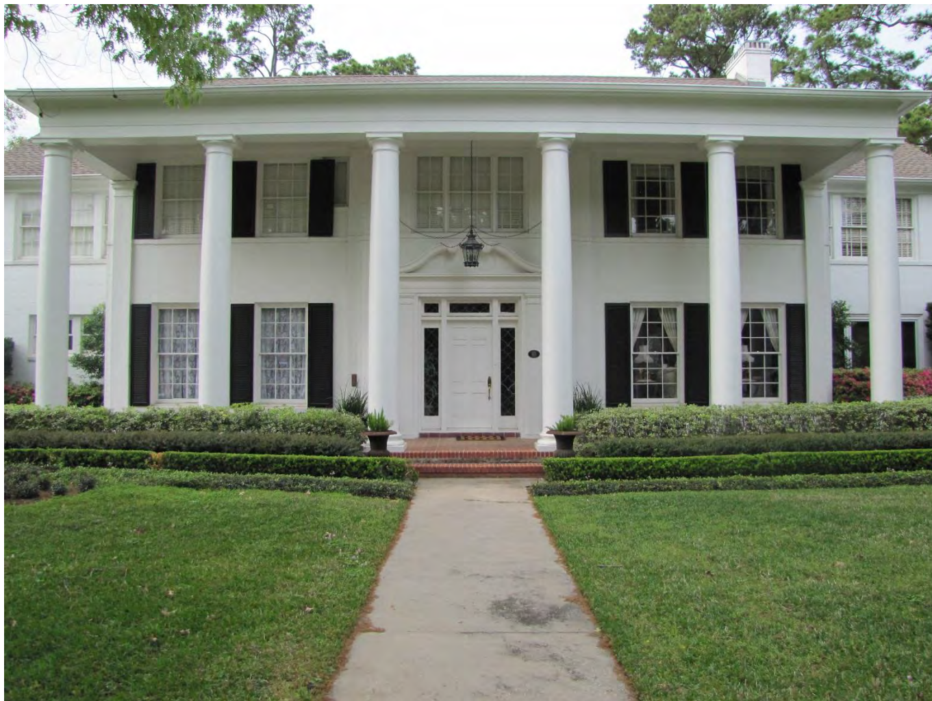
Photo 2: Primary (south) elevation showing Neoclassical portico and multi-pane double-hung sash windows. Camera facing north.
