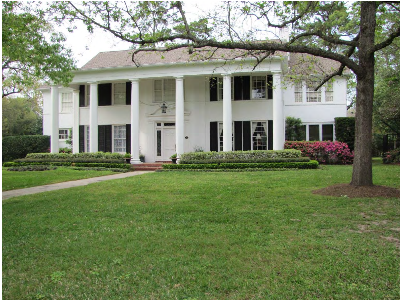
Photo 12: Primary (south) elevation. Camera facing northwest.
