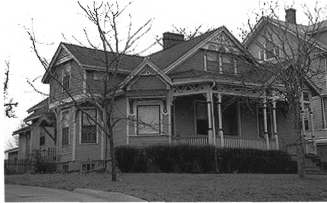
528 Oakland Avenue - Cross Gabled Cottage (Queen Anne)
