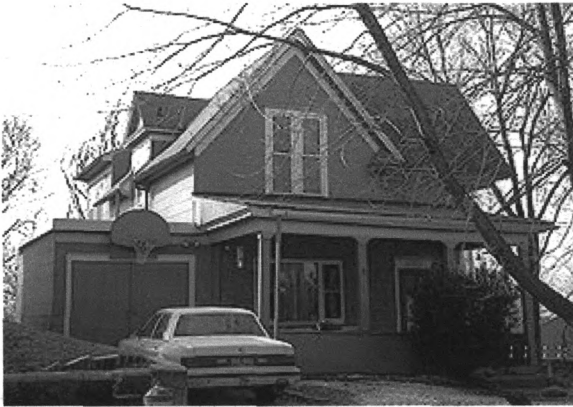
333 Lawton Terrace - Cross Gabled Cottage
