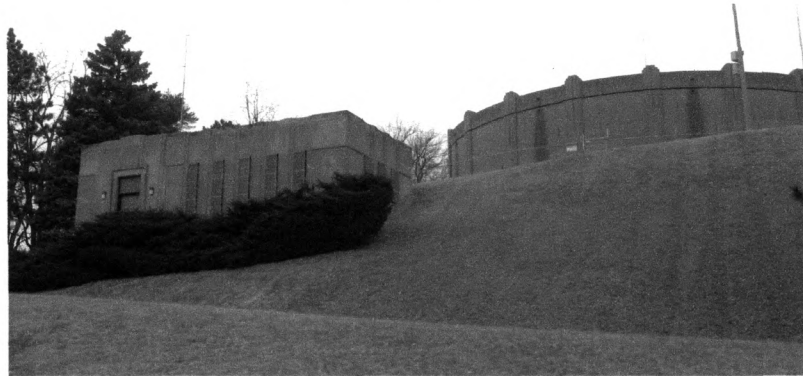
Council Bluffs Waterworks on Lawton Terrace - Modernistic
