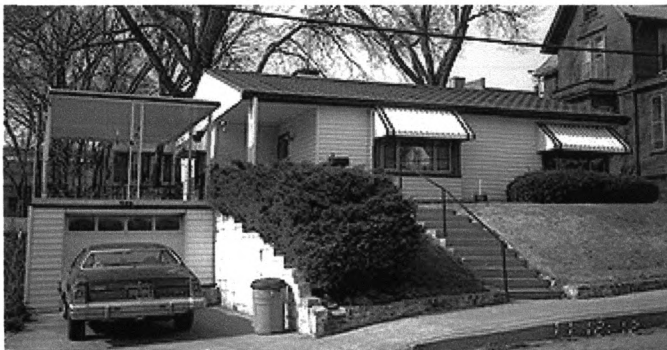
222 N. 2nd Street - Lustron House (with cover-up siding)
