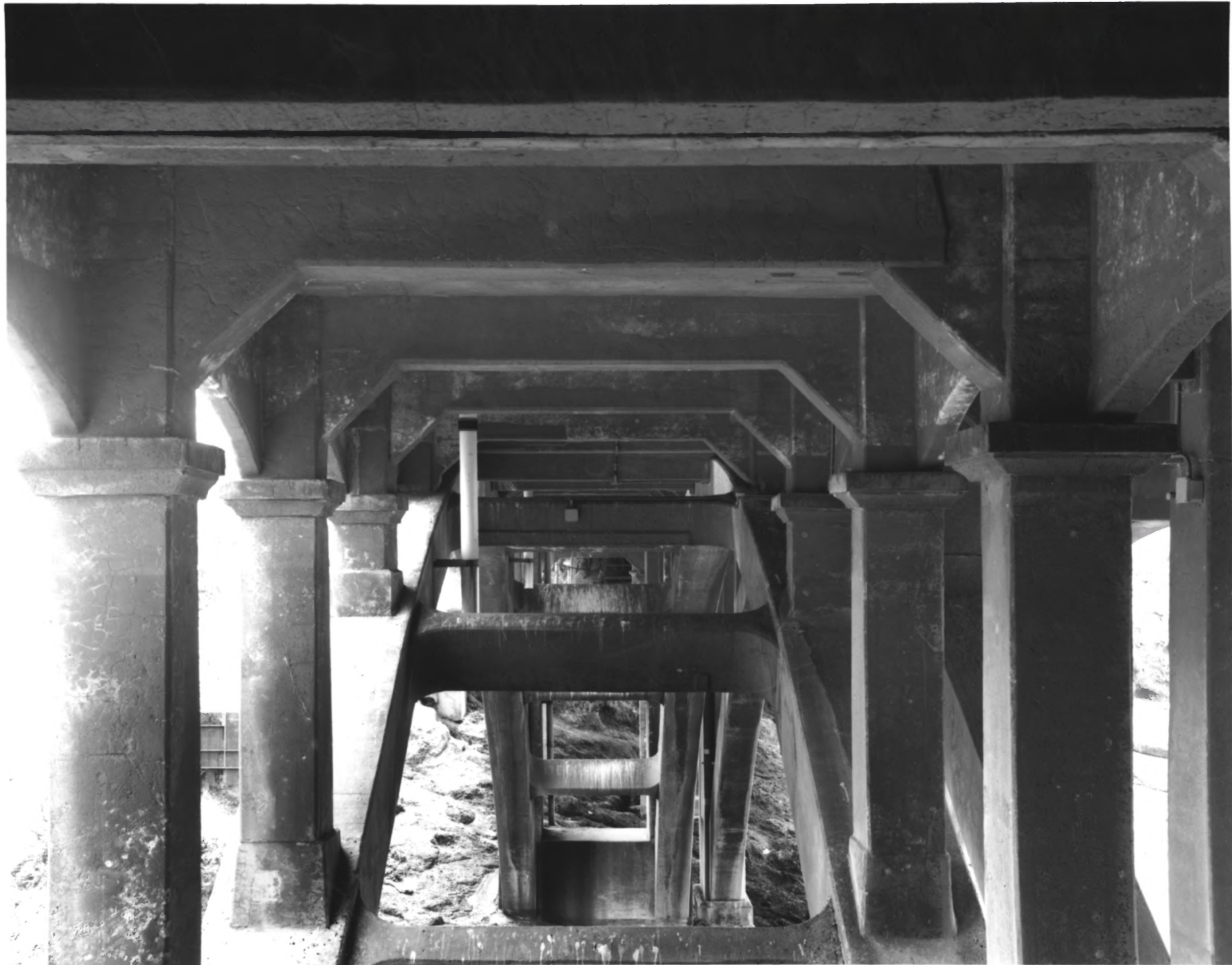
DEPOE BAY BRIDGE, DEPOE BAY, OREGON
