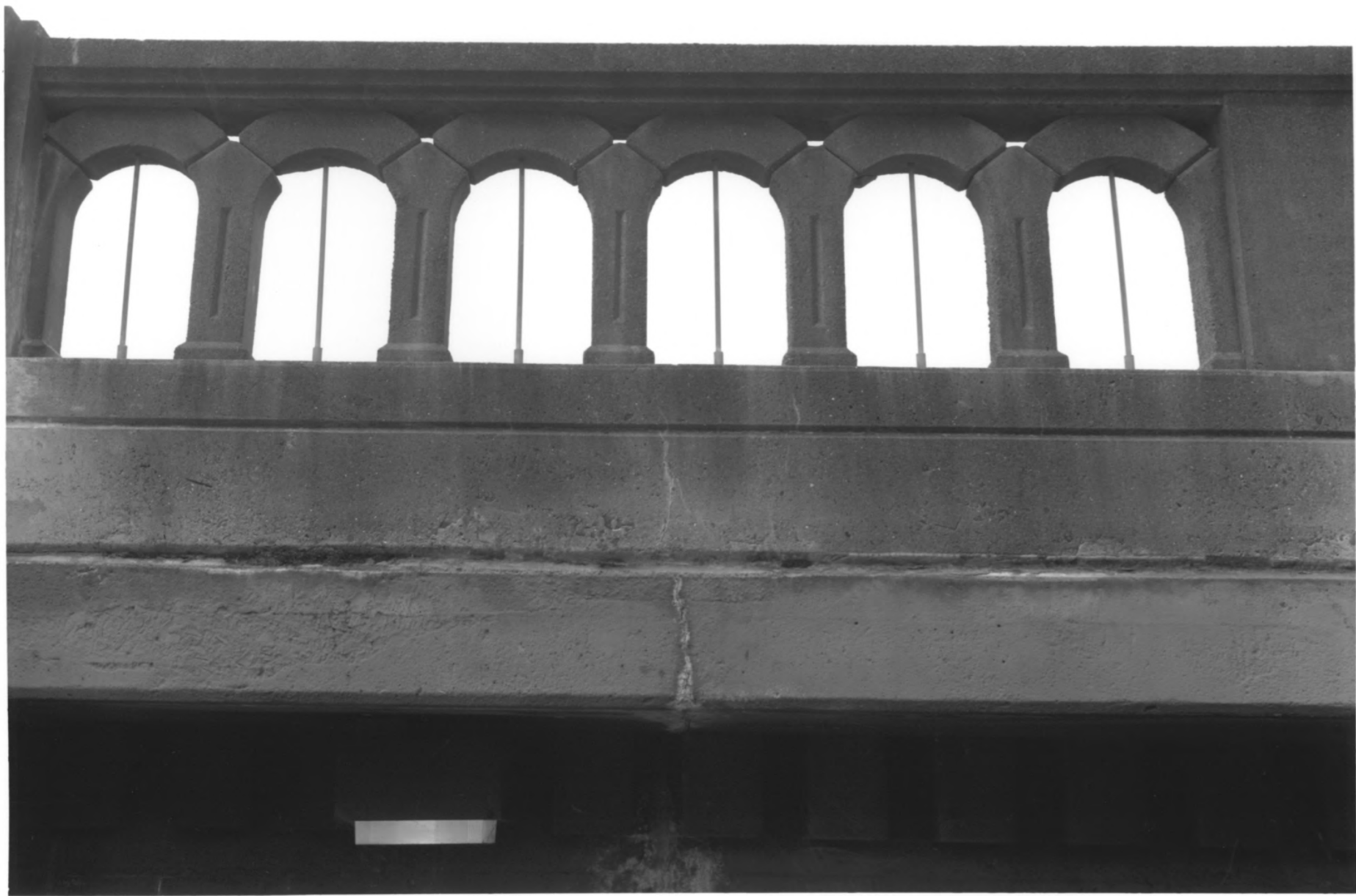
DEPOE BAY BRIDGE, DEPOE BAY, OREGON
