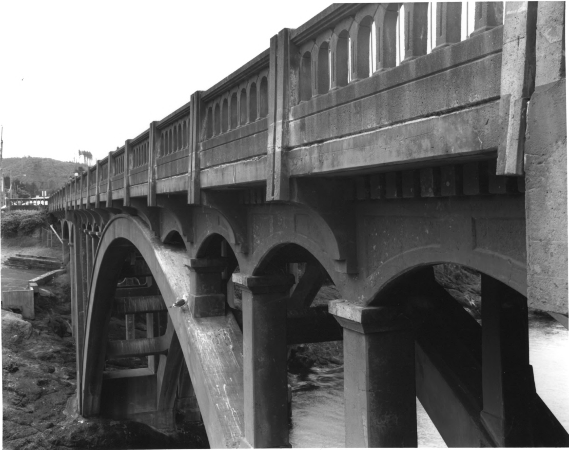
DEPOE BAY BRIDGE, DEPOE BAY, OREGON # 5
