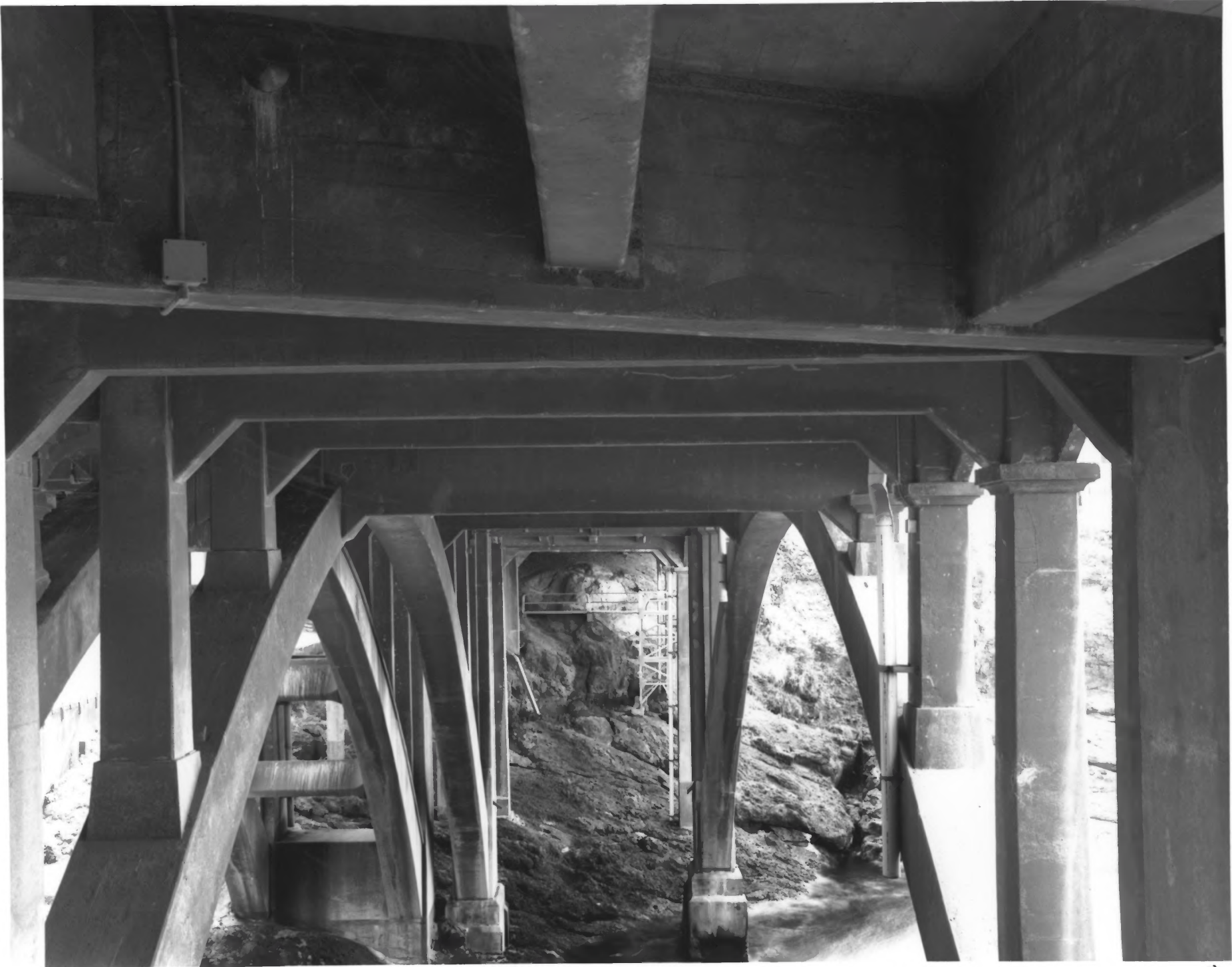
DEPOE BAY BRIDGE, DEPOE BAY, OREGON
