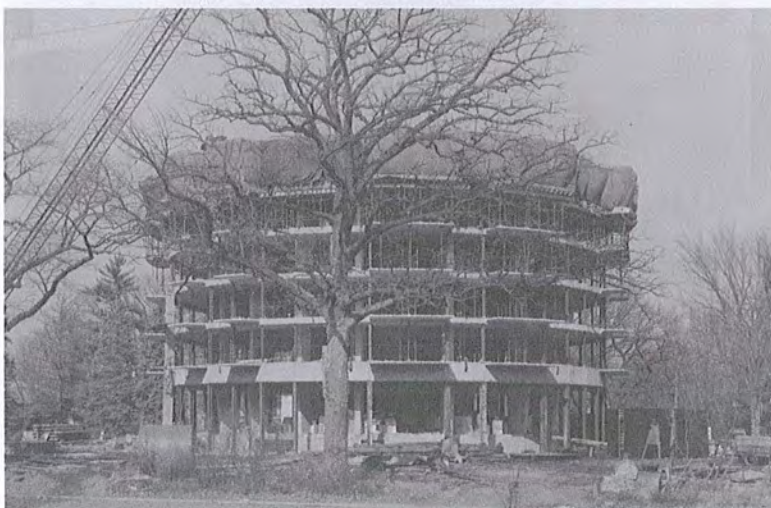
(SOURCE: Plymouth Place – Construction files.)
