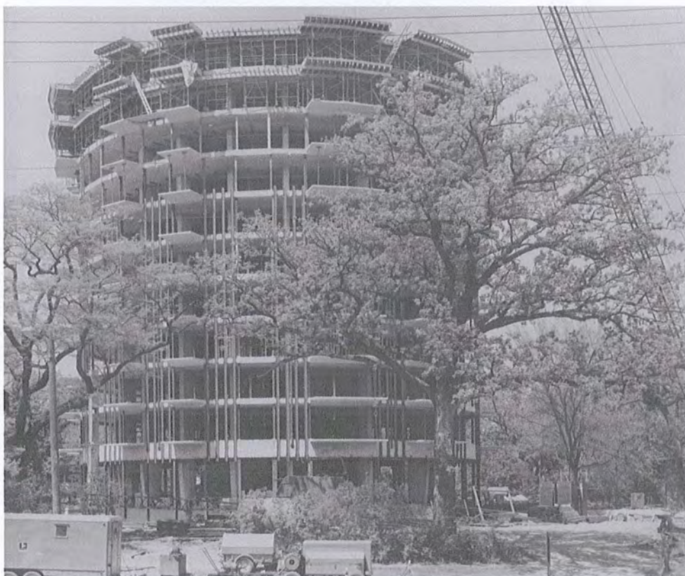
Figure 8. Construction Photo (May 1967)
