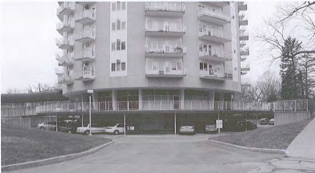
Figure 10. Photograph (Image 0003) – View of Concrete Terrace and Ground Level Parking
