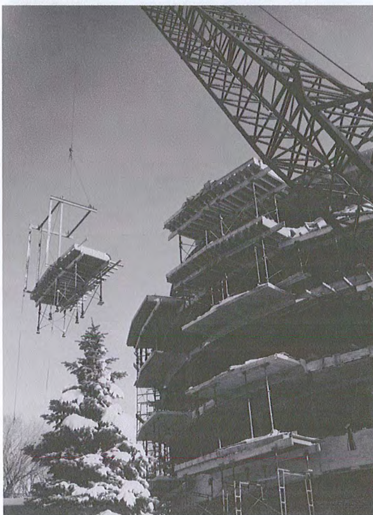
Figure 9. Construction Photo (May 1967)
