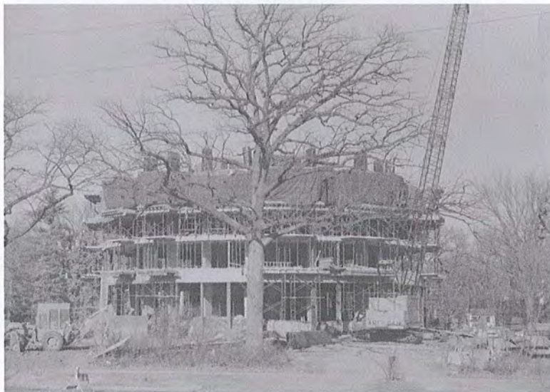
(SOURCE: Plymouth Place – Construction files.)
