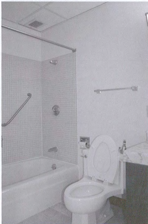
Figure 18. Photograph (Image 0014) – Typical Bathroom on Floors 2-12
