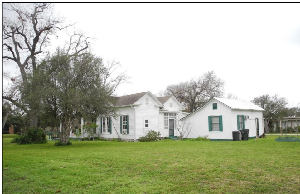
PHOTO 4: King-Woods House (rear) and Kitchen/Smokehouse, east and north elevations, facing southwest (February 1, 2017).
