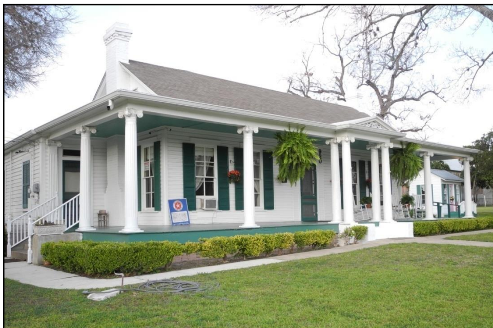
PHOTO 2: King-Woods House, west and south elevations, facing northeast (February 1, 2017).
