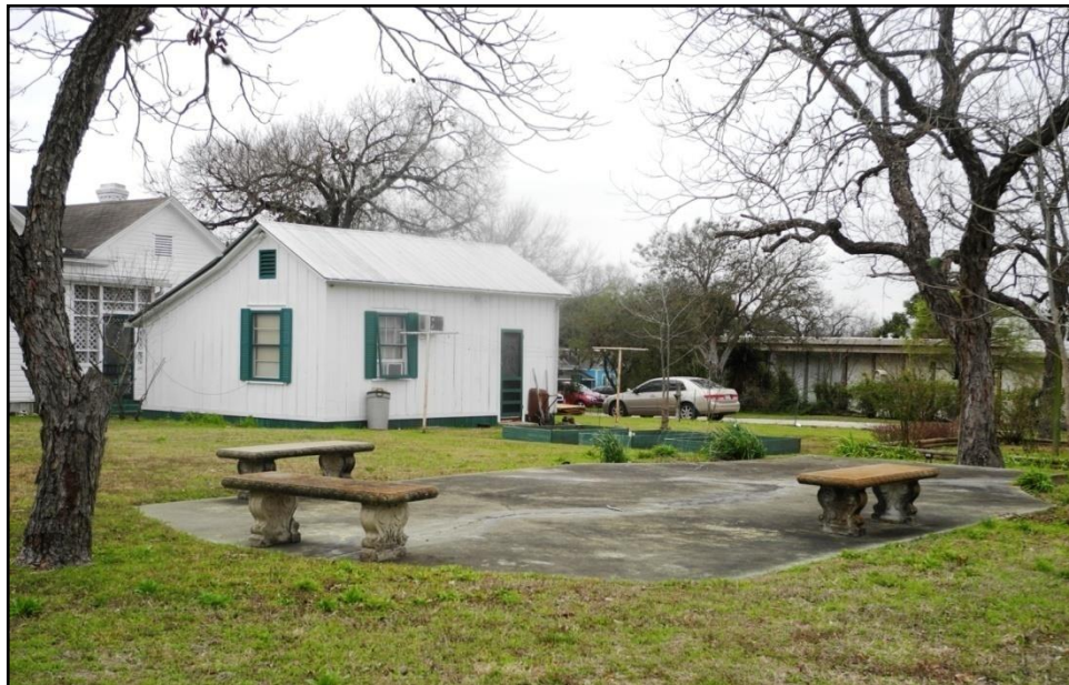
PHOTO 17: King-Woods Kitchen/Smokehouse, east and north elevations, facing southwest (February 1, 2017).
