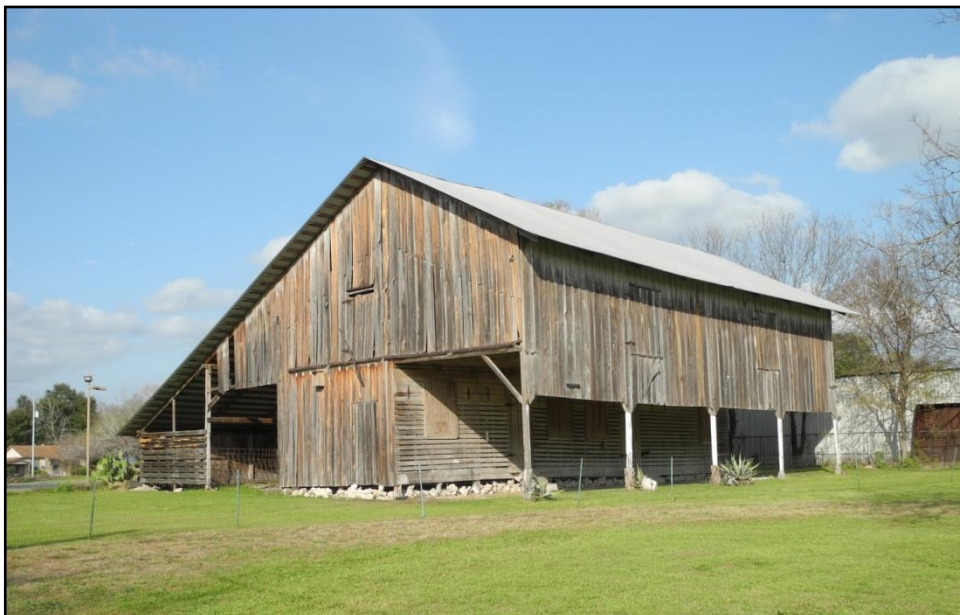
PHOTO 11: King-Woods Multi-purpose Barn, c. 1895, west and south elevations, facing northeast (December 10, 2016).
