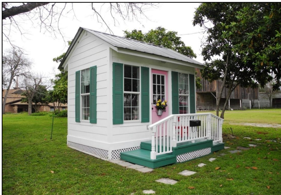
PHOTO 18: King-Woods Playhouse, 1947, west and south elevations, facing northeast (April 23, 2017).
