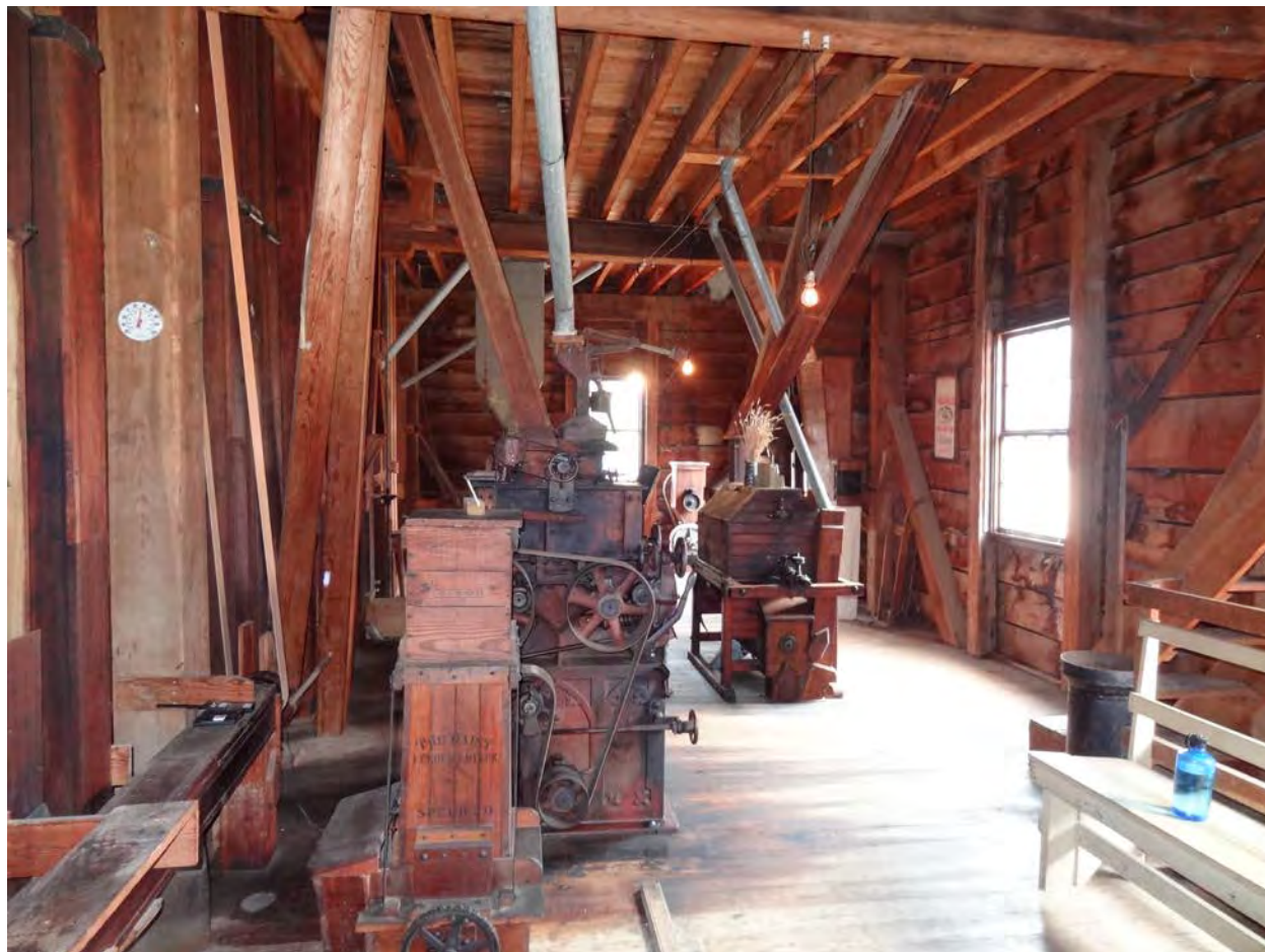
Figure 4: First floor, machinery, including feeder/mixer built by Barnard and Leas Manufacturing Company, roller mill built by Barnard and Leas Manufacturing Company, and bran duster built by Barnard and Leas Manufacturing Company, photograph, January 2014, from the files of the Missouri State Historic Preservation Office.
