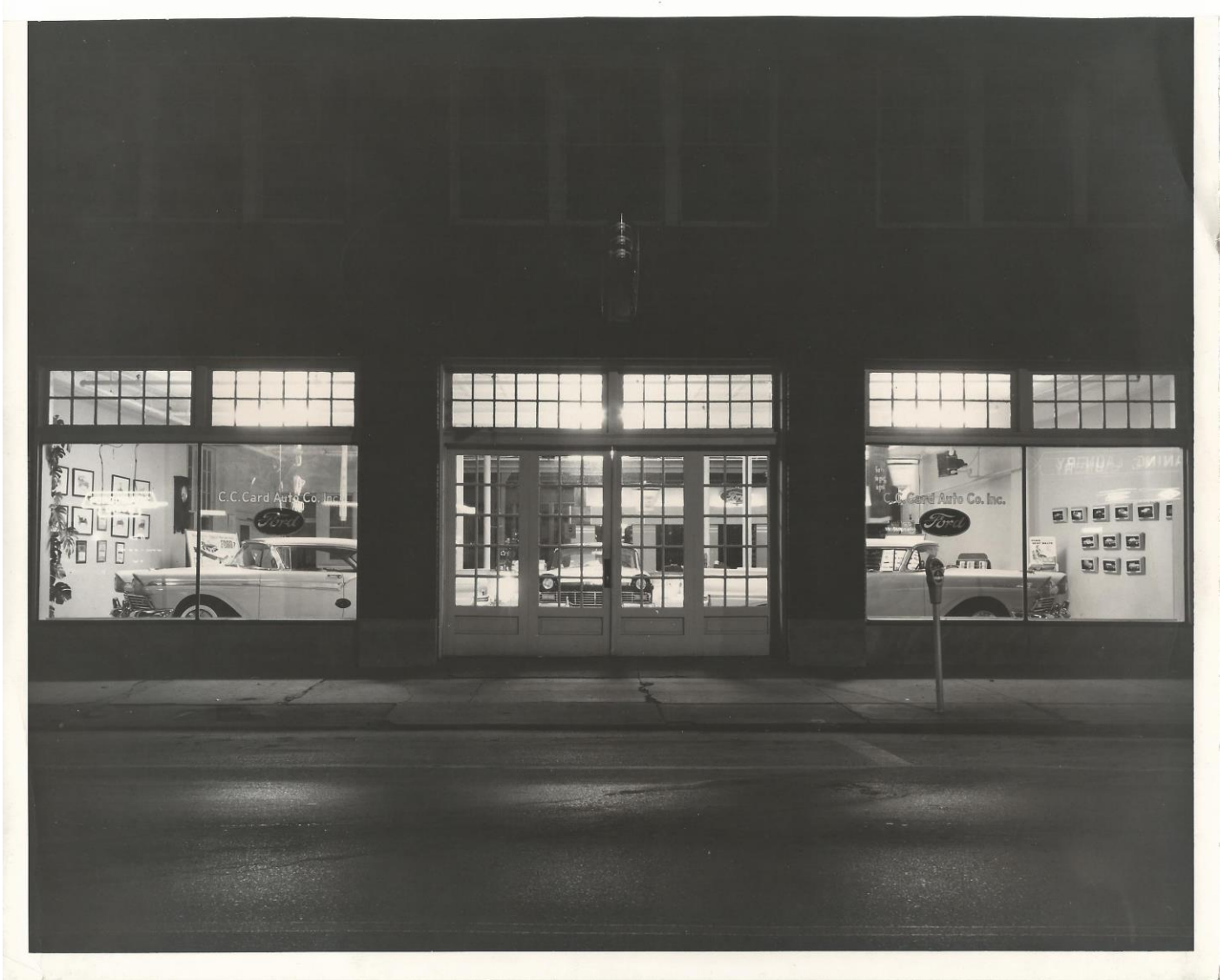
Figure 10. C. C. Card Auto Company showroom, ca. 1950. View north.
