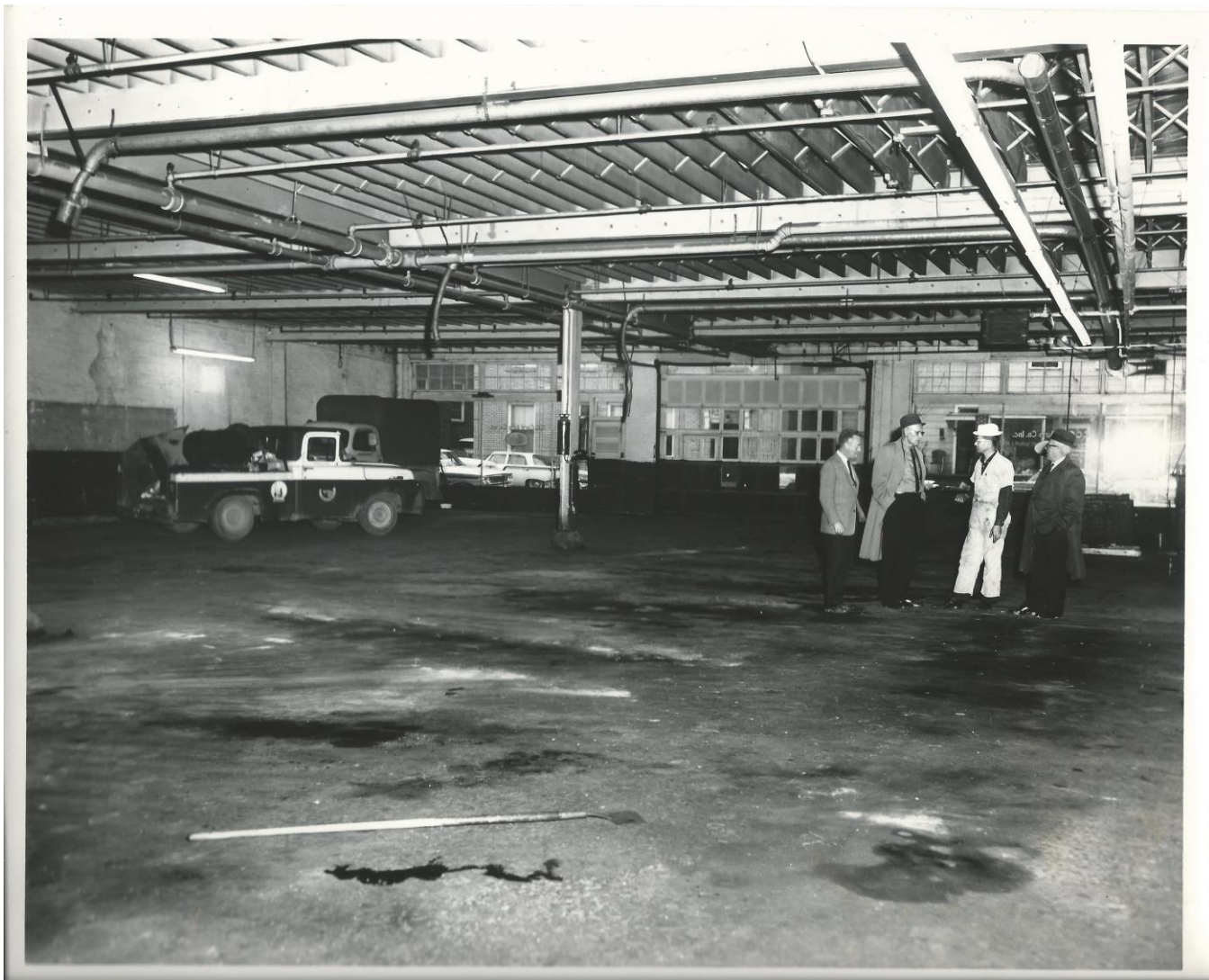
Figure 16. C. C. Card Auto Company, service garage, ca. 1960. View north.
