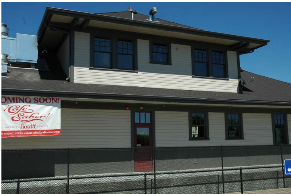
Photograph 6 West elevation detail. Camera facing northeast.
