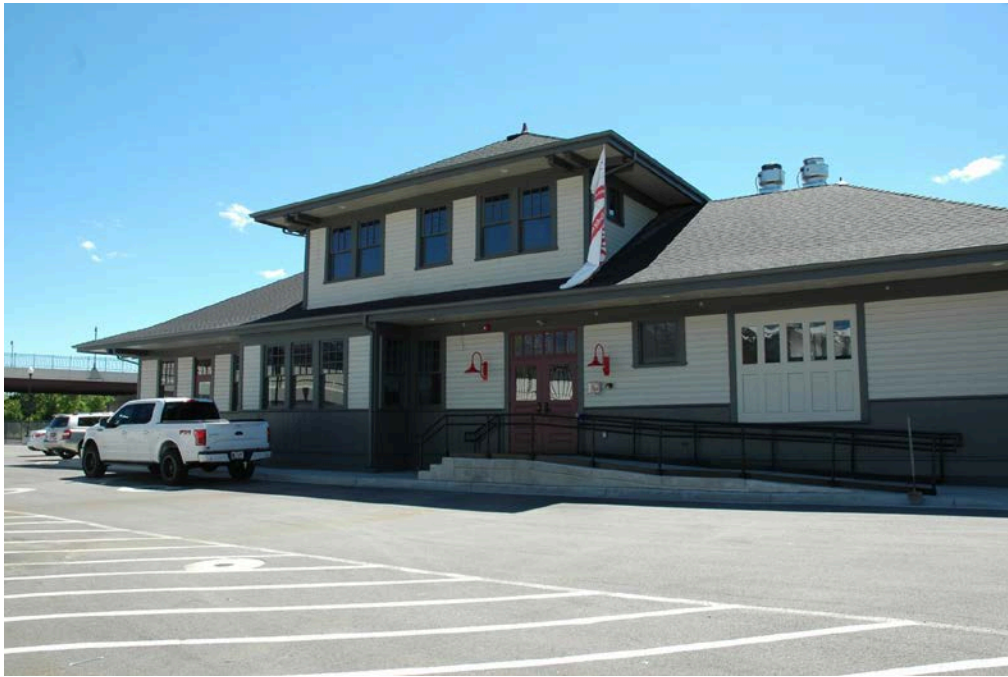
Photograph 1 East elevation of station. Camera facing southwest.
