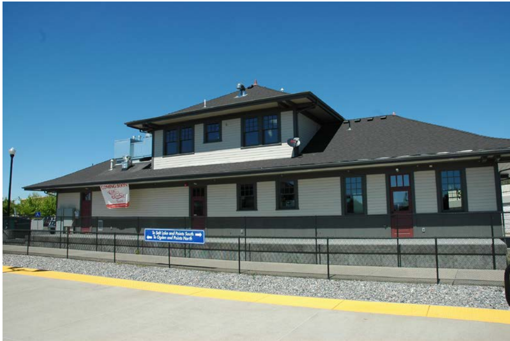
Photograph 5 West elevation. Camera facing northeast.
