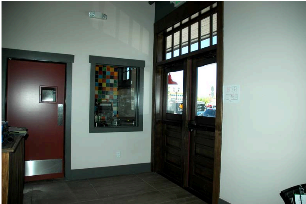
Photograph 7 Interior, main floor, east entry. Camera facing north.
