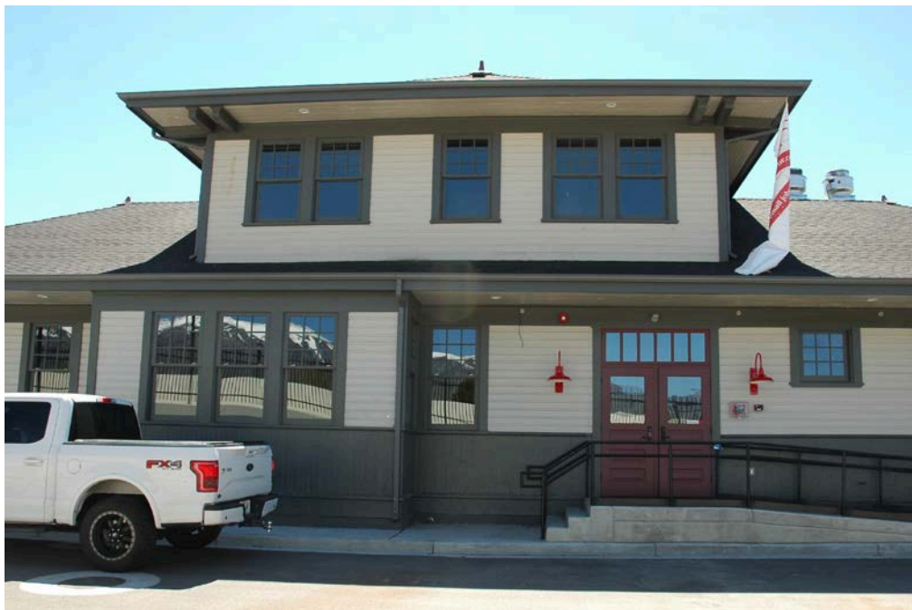
Photograph 2 East elevation, entrance. Camera facing southwest.
