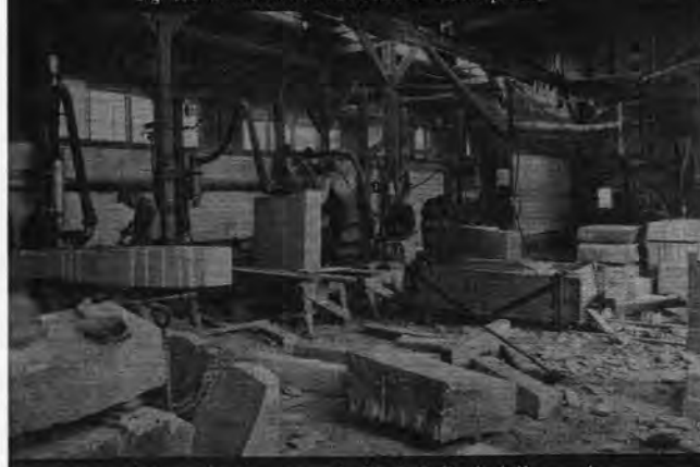
One of the modern high-speed polishers shown in the recent well-lighted addition to the Beck & Beck plant.
