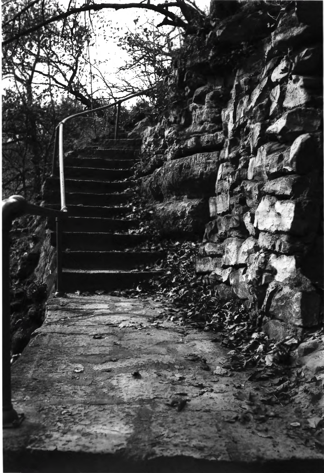
MINNEOPA STATE PARK BLUE EARTH CO., MN STRUCTURE #7, PHOTO I.P. 09344 #15
