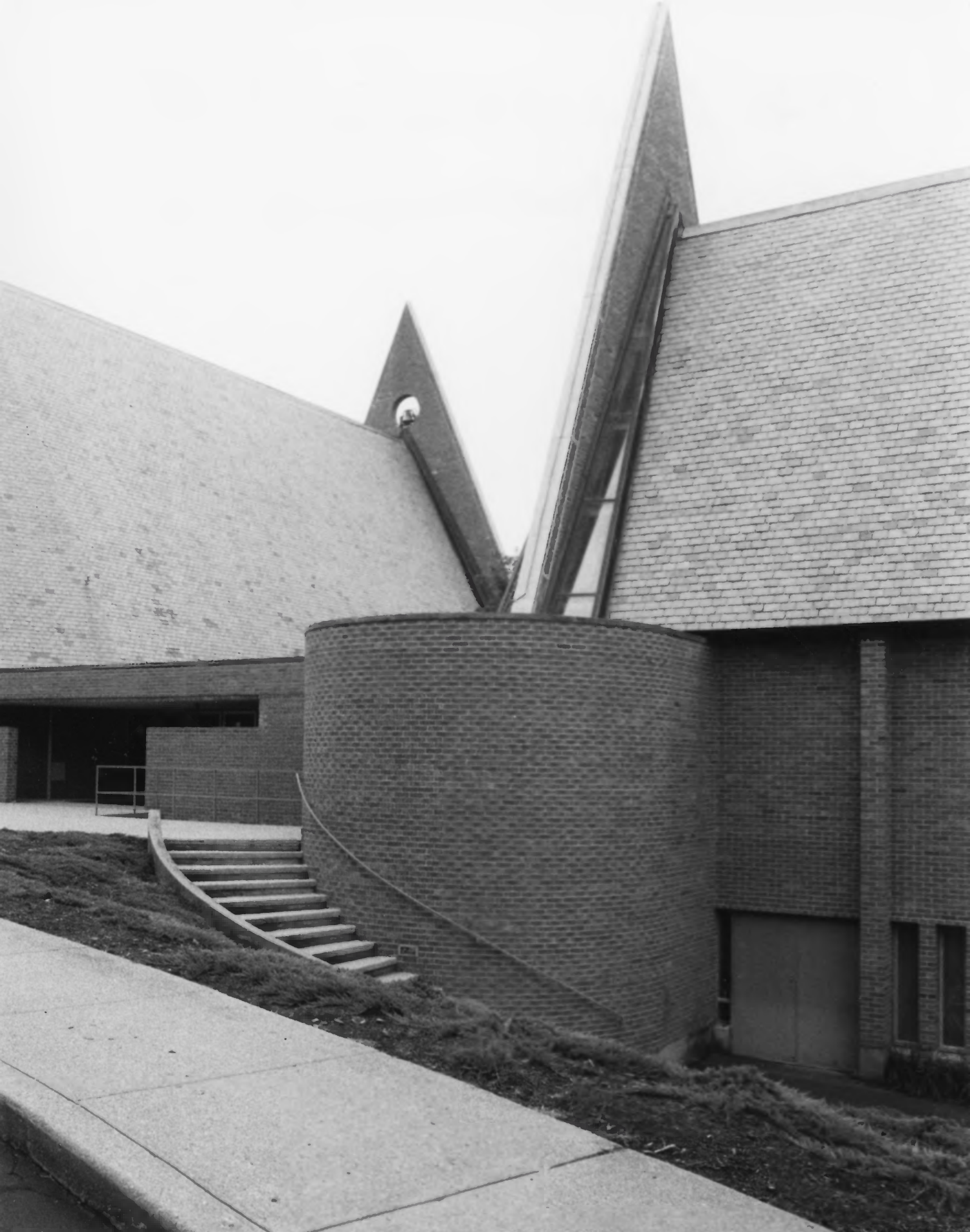
FIRST BAPTIST CHURCH Columbus, Indiana Detail of north facade Photo: Historic Landmarks Foundation of Indiana Inc., 1999
