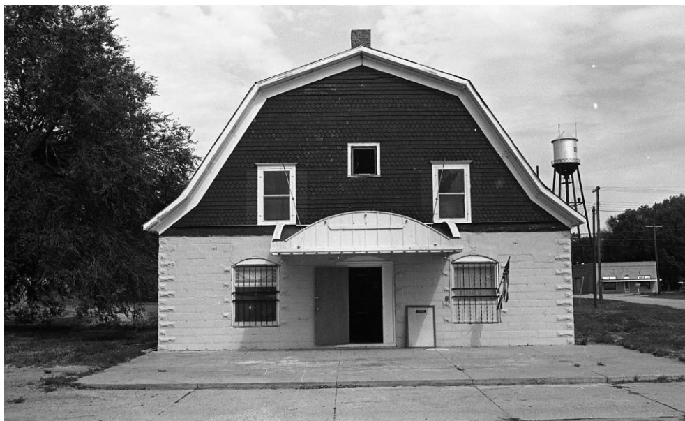
Figure 2: Oshkosh Opera House (GD03-001) with Oshkosh Water Tower featured in the background; looking east, 1975 (Nebraska SHPO site files).
