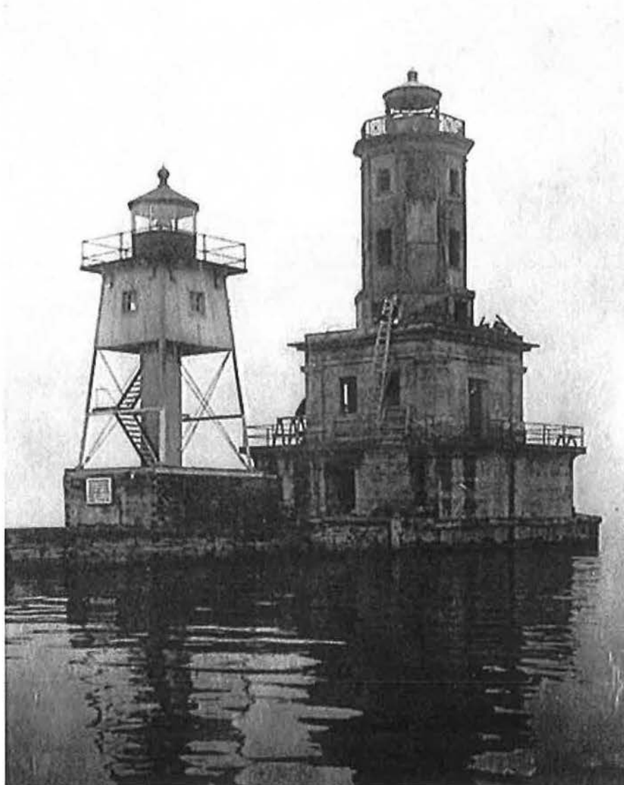
Figure 2. Historic Photograph. This 1920 photo shows the Keweenaw Waterway Lower Entrance Light under construction and the 1911 Portage River Pierhead Light, camera facing southeast. Photographer: Unknown. Location of original photo: Record Group 26, National Archives and Records Administration.
