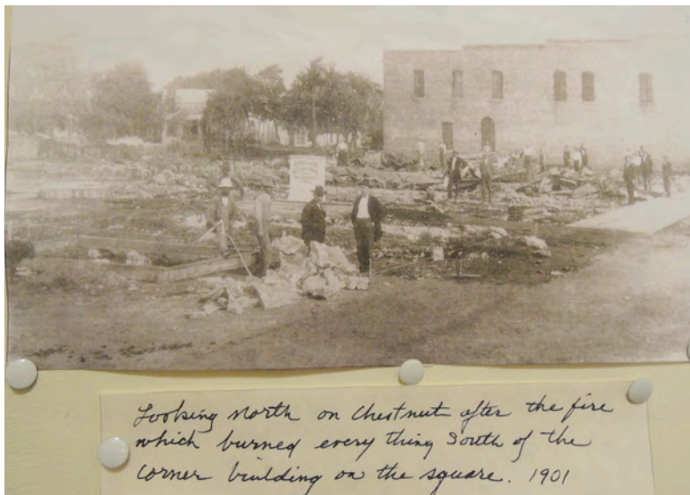
Figure 9: Photograph from 1901 showing Bricker-Price Block (arrow) still standing after destructive fire burned all commercial buildings to the south. (Courtesy Earlham Historical Society Museum)
