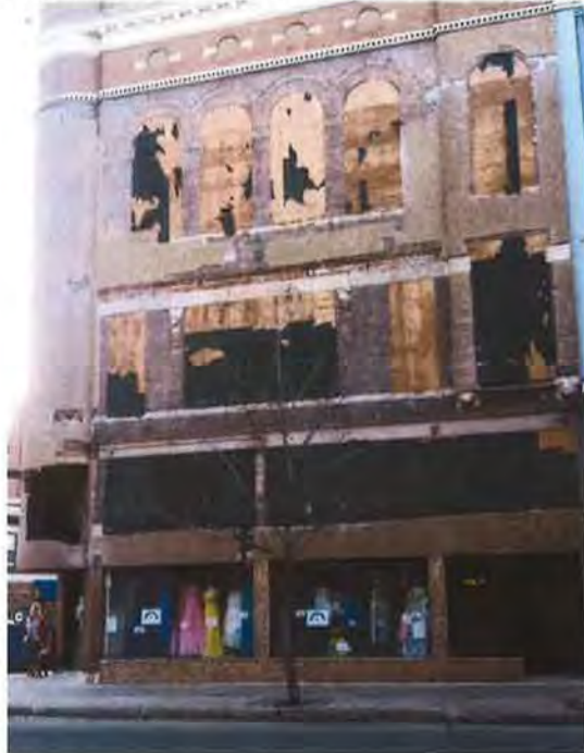
Appearance, January 2016, after removal of stucco covering:
