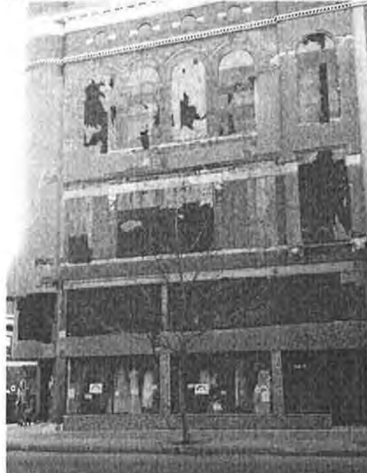
Appearance, January 2016, after removal of stucco covering:
