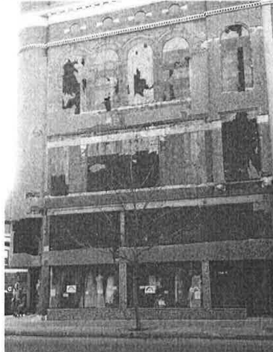
Appearance, January 2016, after removal of stucco covering:
