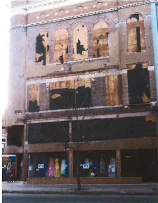
Appearance, January 2016, after removal of stucco covering:
