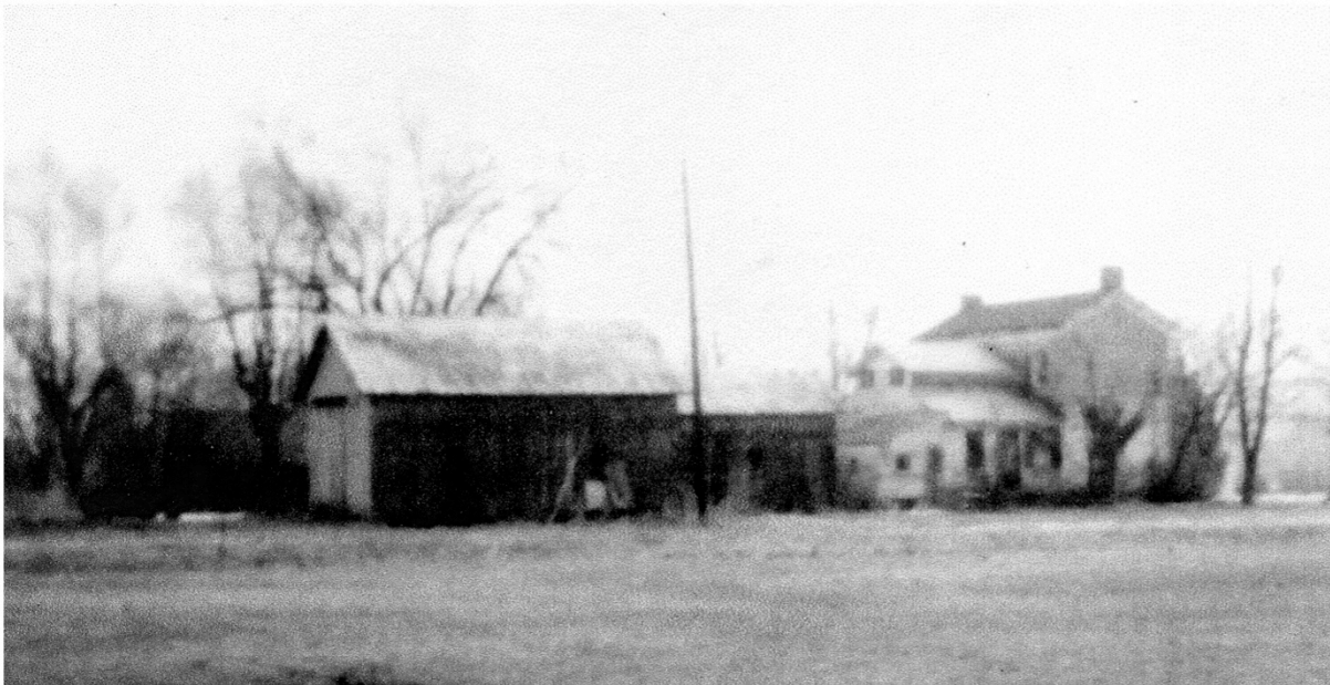
Figure 3: View of 1841 House and old additions, taken in 1976. Photo given to Decker family by visitors to property in 1983.
