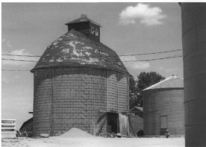
Figure 8 Double bin, concrete block corn crib. (Tallgrass Historians L.C., 2007)
