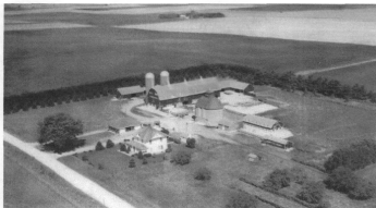
Figure 5 Aerial view of Tyden Farm No. 6, circa 1940s. All buildings are thought to have been constructed by Tyden except the farmhouse and wash house. Except for the clay tile silos and a smaller wooden machine shed beside them, all these buildings are extant. (Courtesy Ted and Judy Pitzenberger, Dougherty, Iowa)
