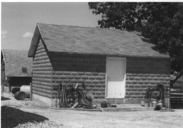
Figure 9 Rock-face concrete block feed shed. (Tallgrass Historians L.C., 2007)
