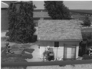
Figure 4 The white-painted wash house (summer kitchen), seen here in the center foreground, appears to date to the same period as the farmhouse itself. Behind and to the left of the frame building stands the vine-covered concrete water storage tank, no longer used. The rock-face concrete block feed shed is visible over the ridge of the wash house, behind the water tank. The two concrete structures are thought to date to Emil Tyden's ownership period. This photograph was taken from the balcony outside the bedroom wing occupied by Tyden during his frequent visits to oversee his farm properties. (Tallgrass Historians L.C., 2007)
