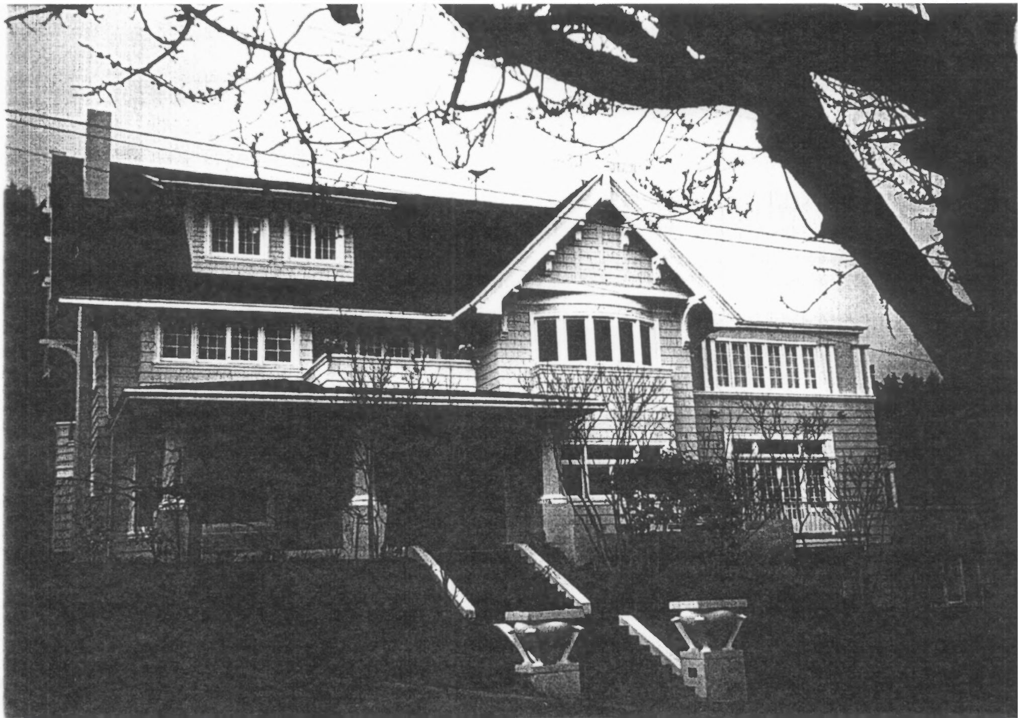
Benefee House, 1989 (after renovation)
