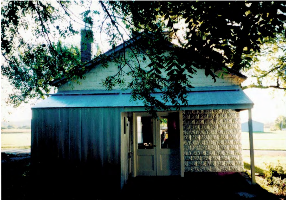
Figure 15. Store, east elevation and porch of, camera facing west
