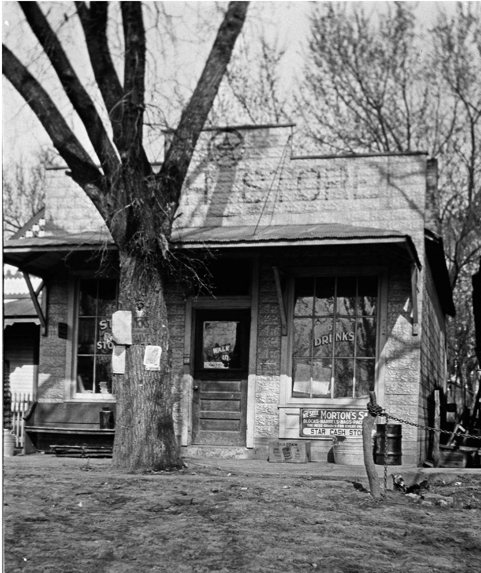
Figure 10. Store, west facade, camera facing east
