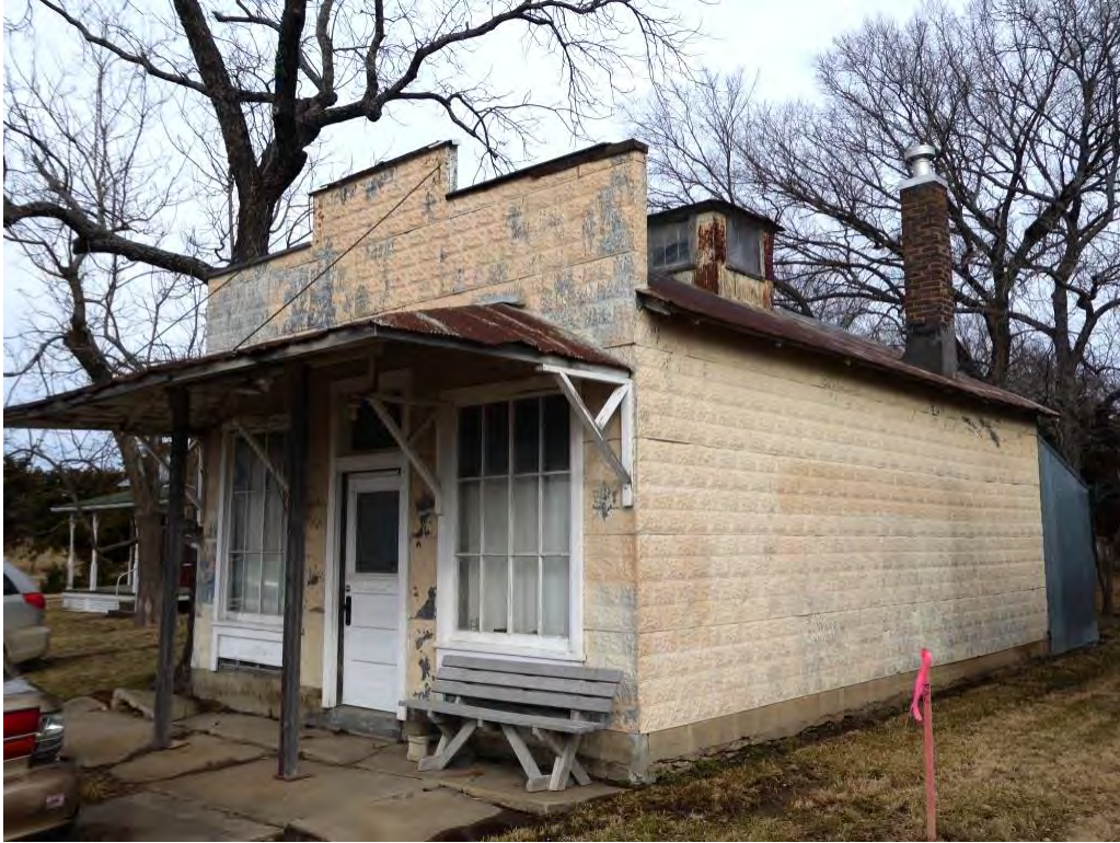
Figure 17. Store, west façade and canopy (left) and south elevation (right) of, camera facing northeast
