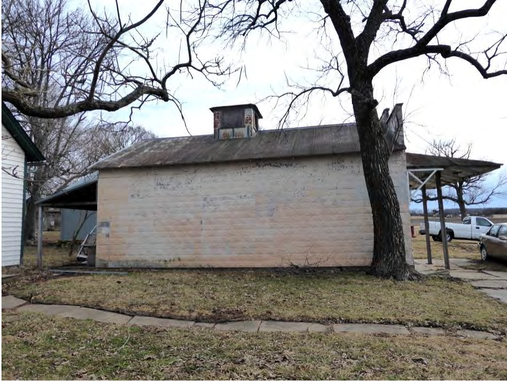
Figure 14. Store, north elevation of, camera facing south
