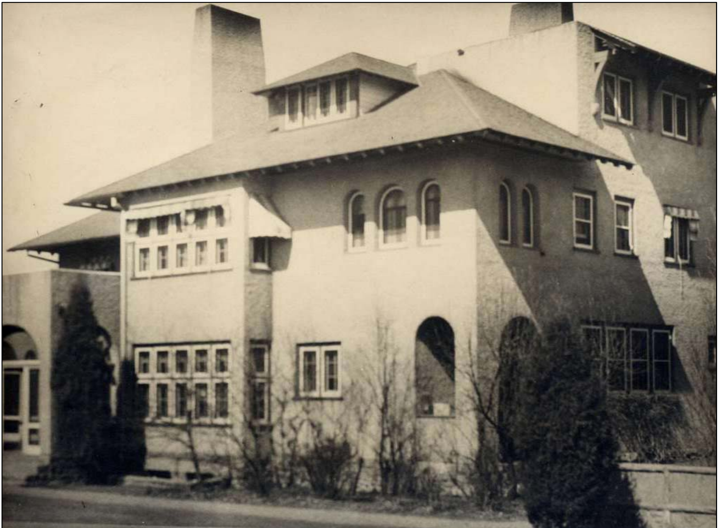
Figure 3. This 1920s or 1930s photograph shows parts of the south and east walls of the house. Courtesy of Tor Hylbom, photographic collection, Arcadia, California.
