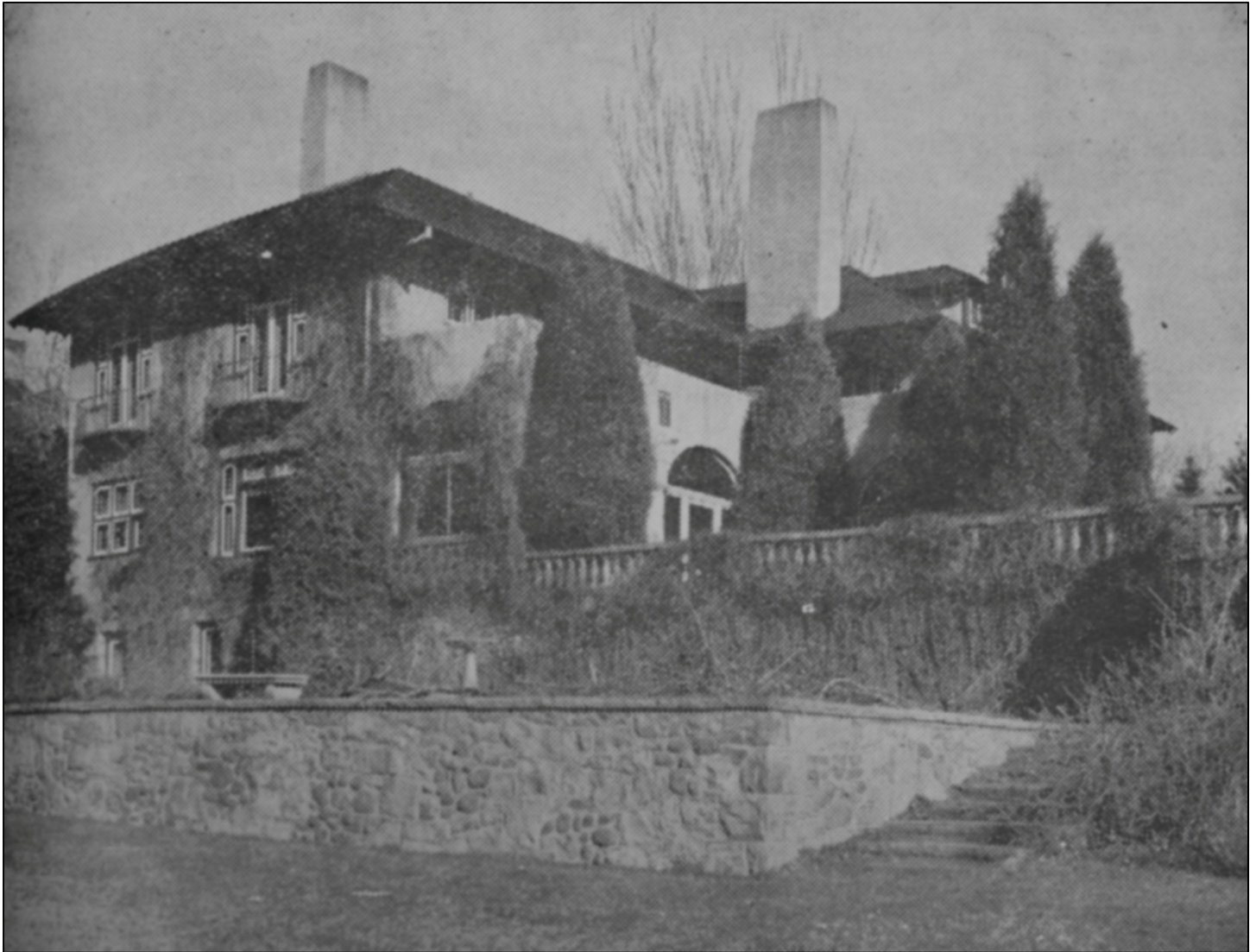
Figure 7. This view northeast shows the property at the time Colorado College acquired it in 1943. The image shows parts of the west and south walls of the house, the parterre on the lower terrace, and the balustrade atop the retaining wall. Courtesy of Colorado College Special Collections, Tiger (Colorado College, Colorado Springs), 2 February 1943.
