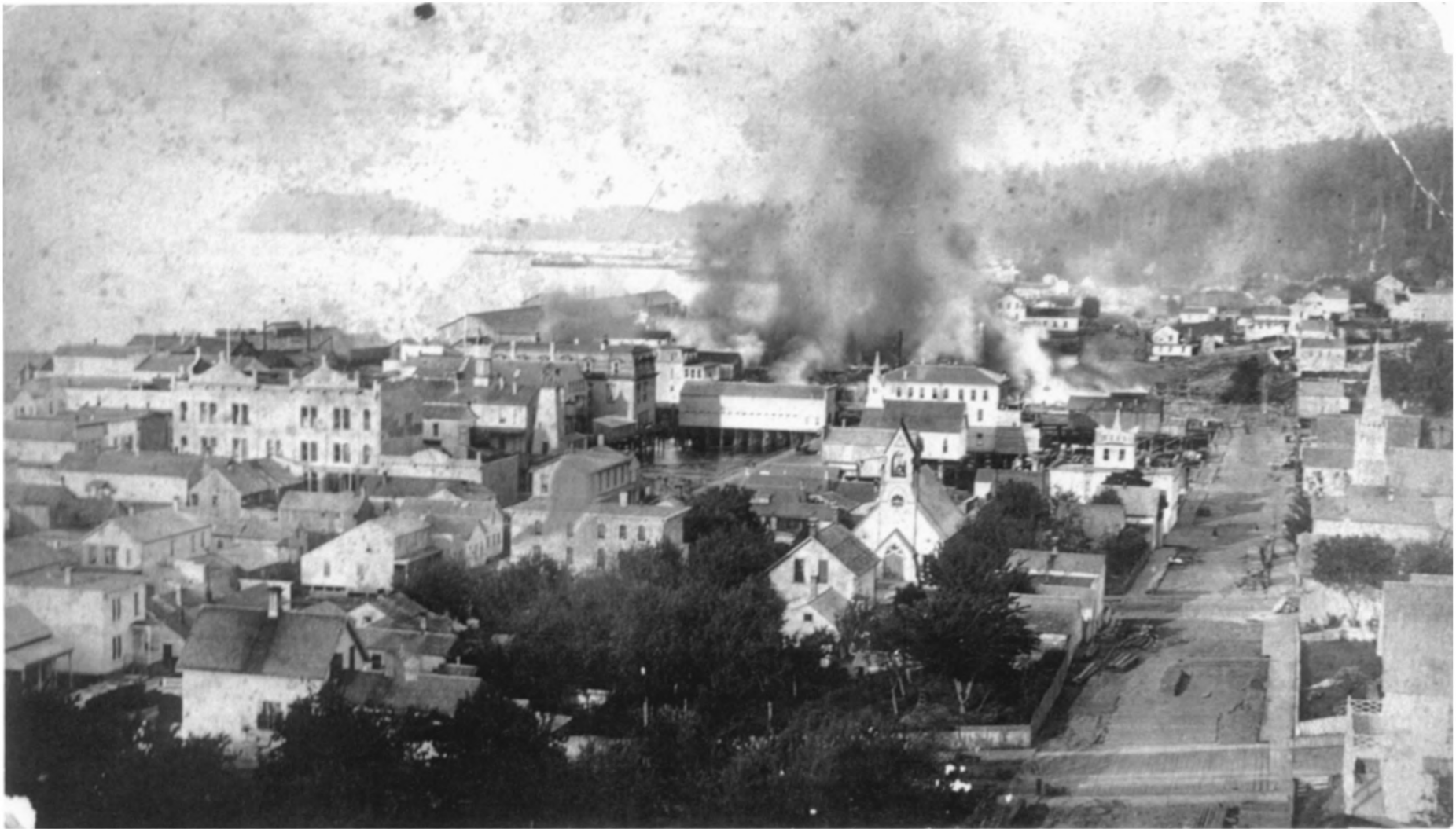
Fig. 21 The fire of 1883, looking east
