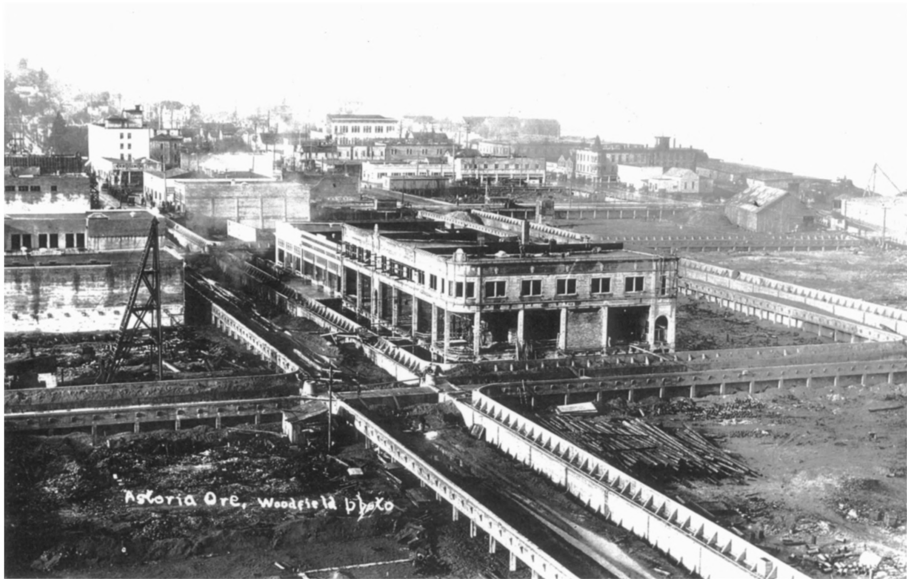
Fig 27 Construction of chairwall, 1923, looking NW courtesy of Art Chan & Bonnie Oathes
