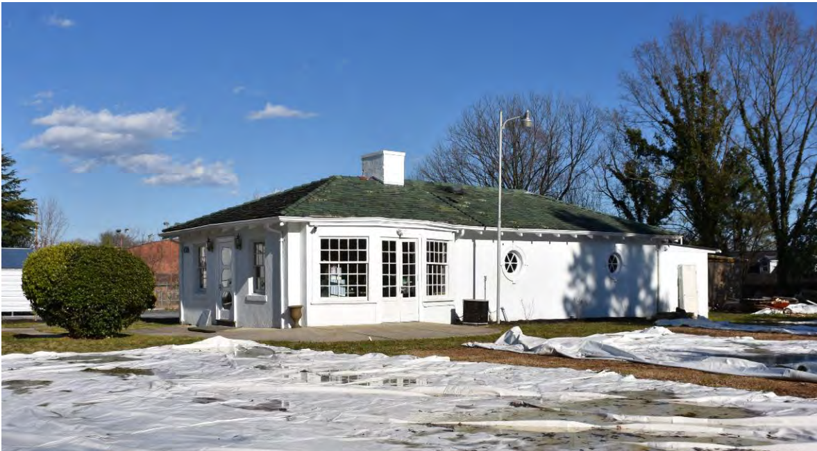
5. Garage, northwest oblique
