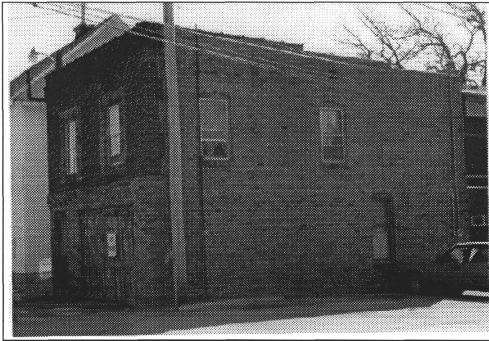
Caretaker's Apartment, Highland Apartments, 606 Euclid Avenue Photograph taken in April, 1996, View to southeast
