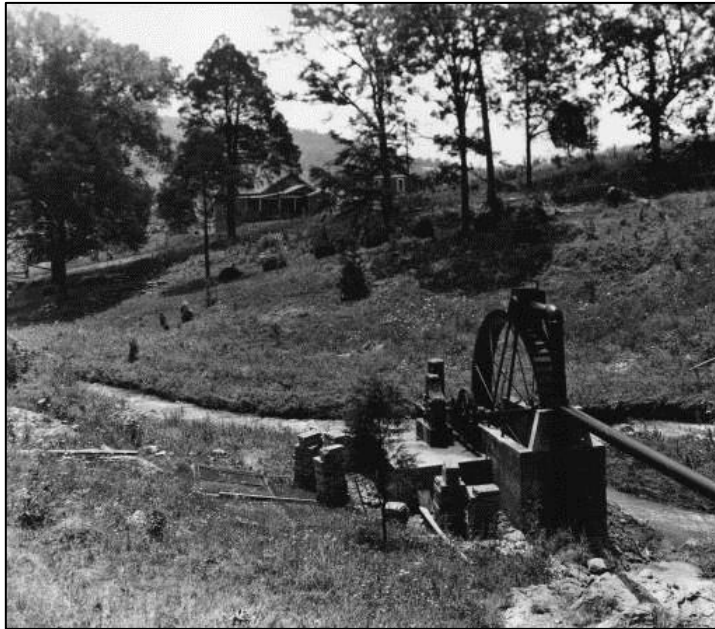
Figure 5: Wheelhouse, Water Wheel and Gatepost ca. 1923 at construction. Photo courtesy of Knox County Public Library: Calvin M. McClung Historical Digital Collection-Thompson Photographic Collection.
