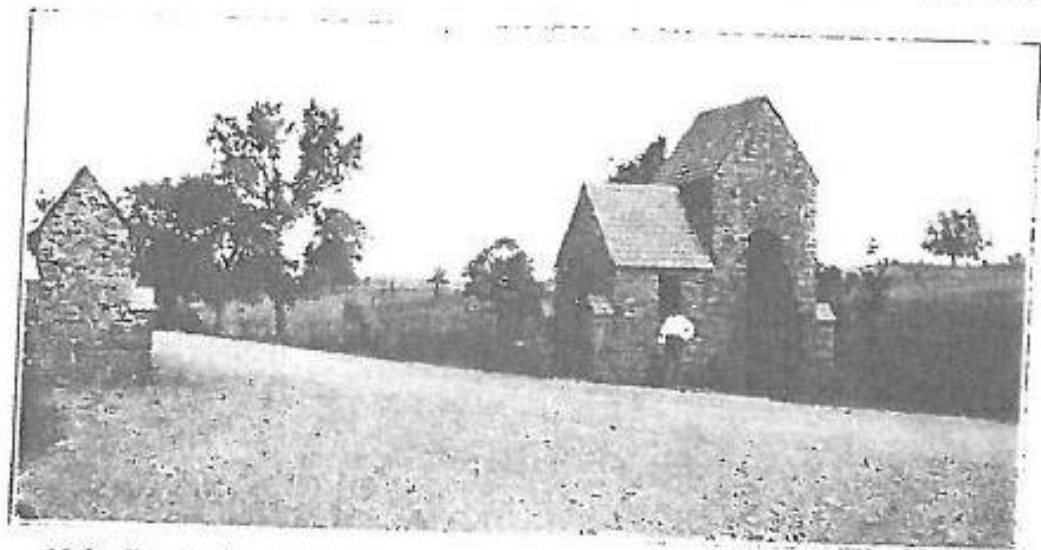
16 ft. diameter by 1 1/4 ft. wide Fitz Water Wheel installed by the Tennessee Mill & Mine Supply Company to operate water supply system for the suburban village of Westmoreland Heights near Knoxville, Tenn. This plant delivers an abundant and unfailling supply of water thru two miles of pipe against a head of 180 ft.
