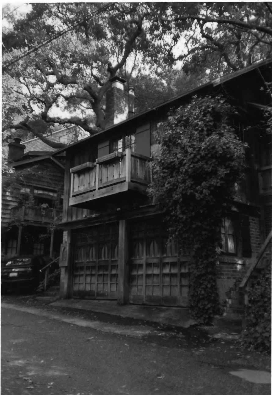
45 Canyon Road, Panoramic Hill, Alameda County, California 31.1(8)
