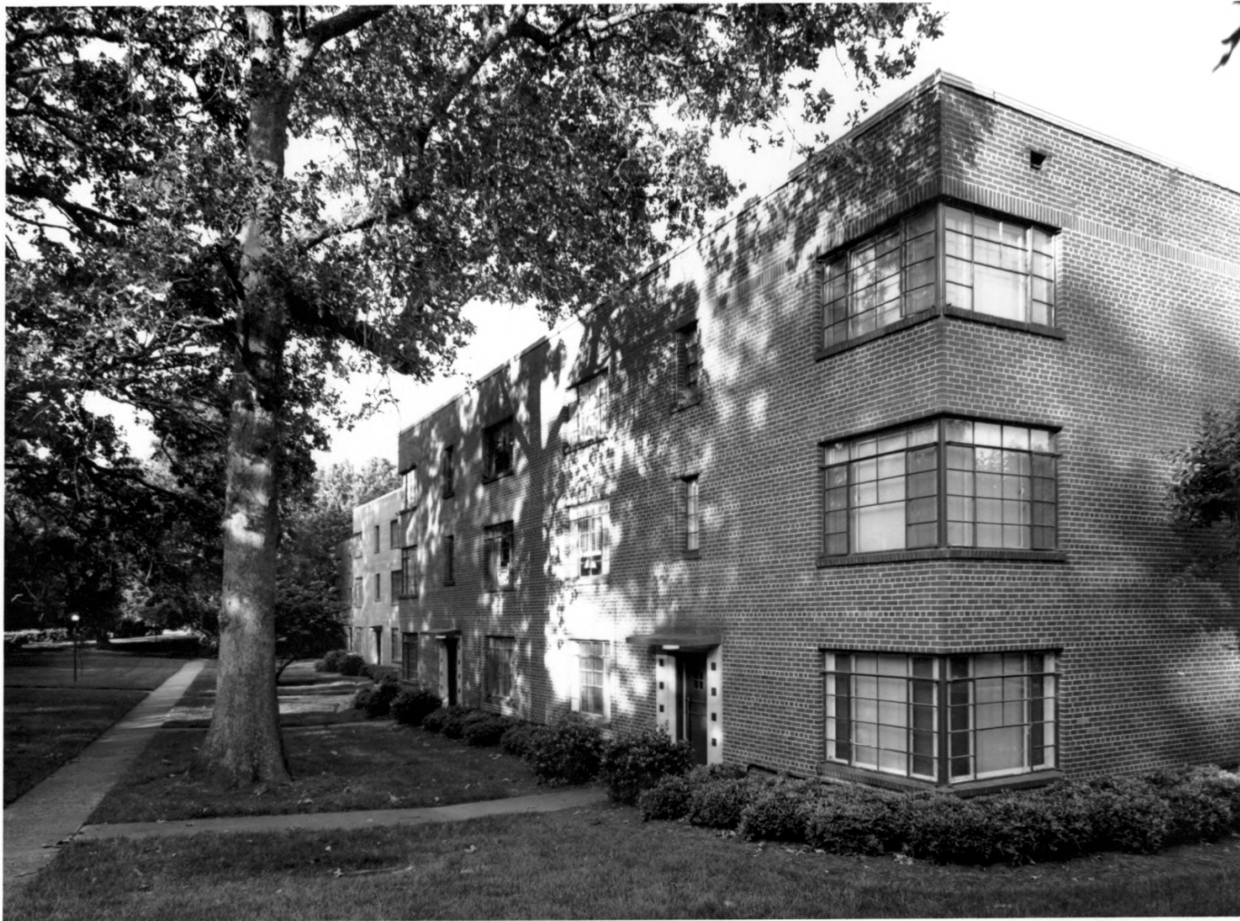
BRIARCLIFF-NORMANDY APARTMENTS D e KALB COUNTY, GEORGIA PHOTOGRAPH 4 OF 23
