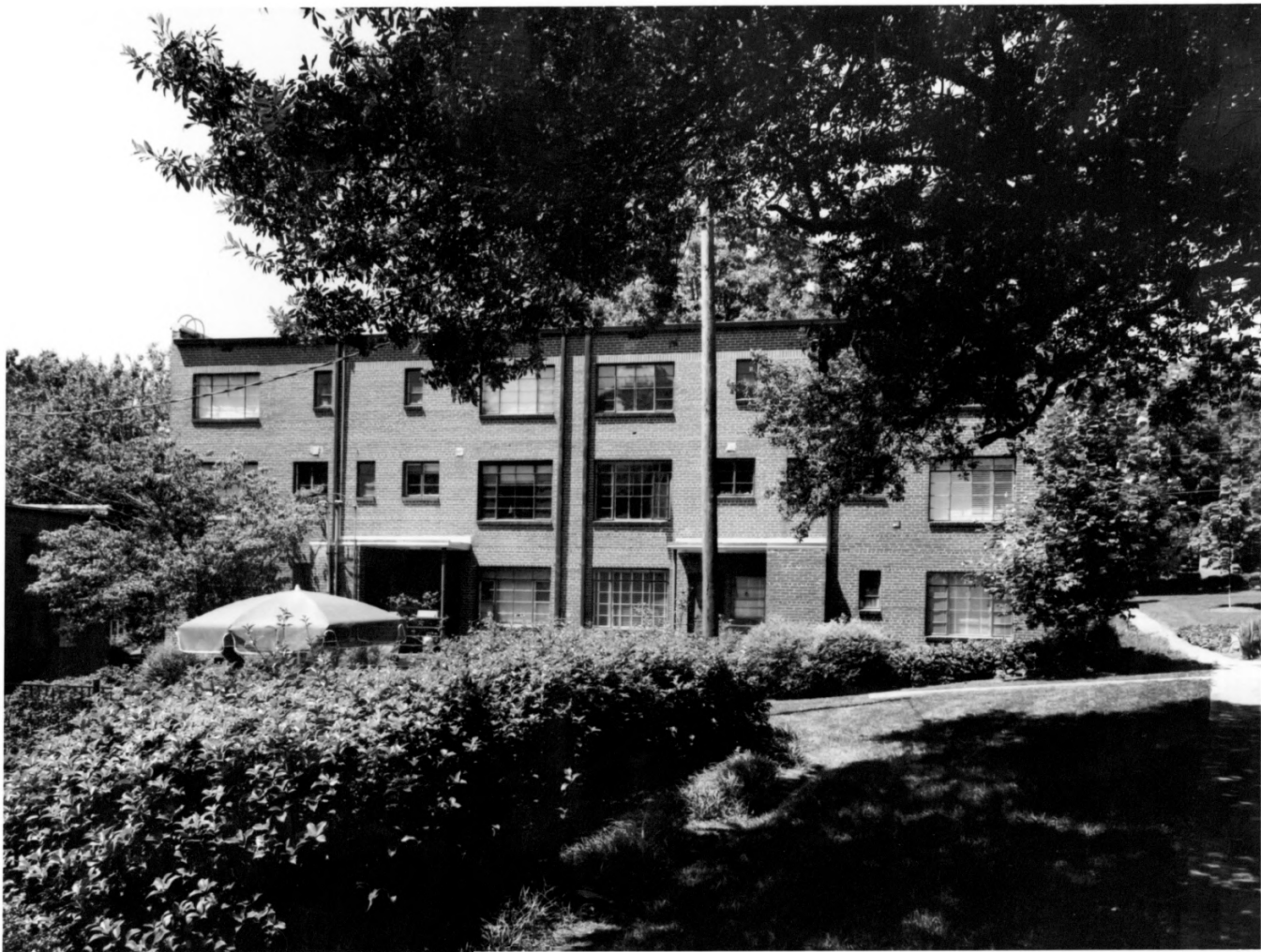
BRIARCLIFF-NORMANDY APARTMENTS D e . KALB COUNTY, GEORGIA PHOTOGRAPH 10 OF 23
