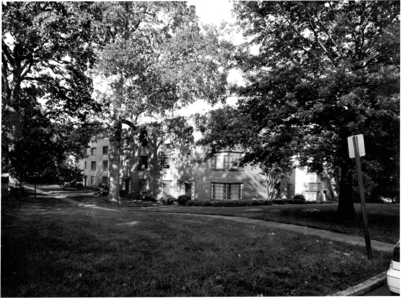
BRIARCLIFF-NORMANDY APARTMENTS D e KALB COUNTY, GEORGIA PHOTOGRAPH 3 OF 23
