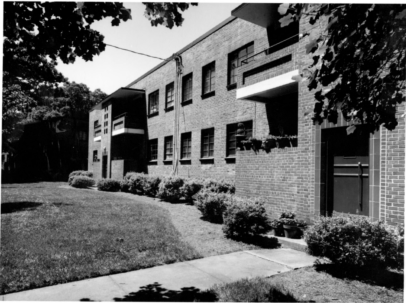
BRIARCLIFF-NORMANDY APARTMENTS D e . KALB COUNTY, GEORGIA PHOTOGRAPH 2 OF 23
