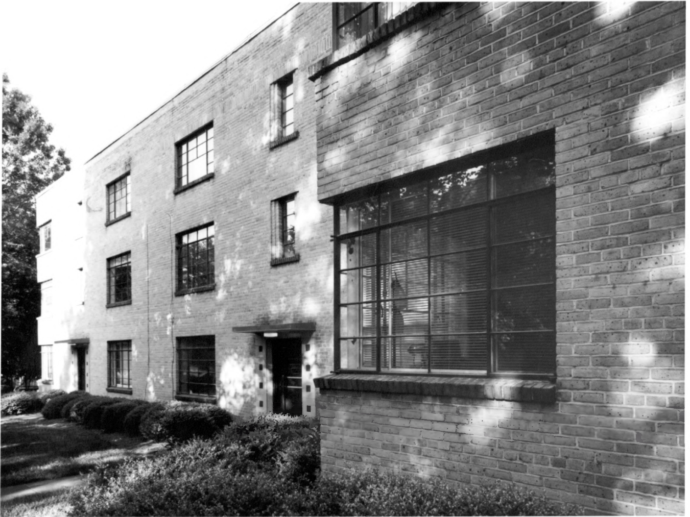
BRIARCLIFF-NORMANDY APARTMENTS D e KALB COUNTY, GEORGIA PHOTOGRAPH 16 OF 23
