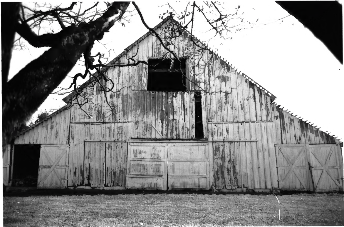
MONDAY HOUSE KNOX COUNTY, TN
