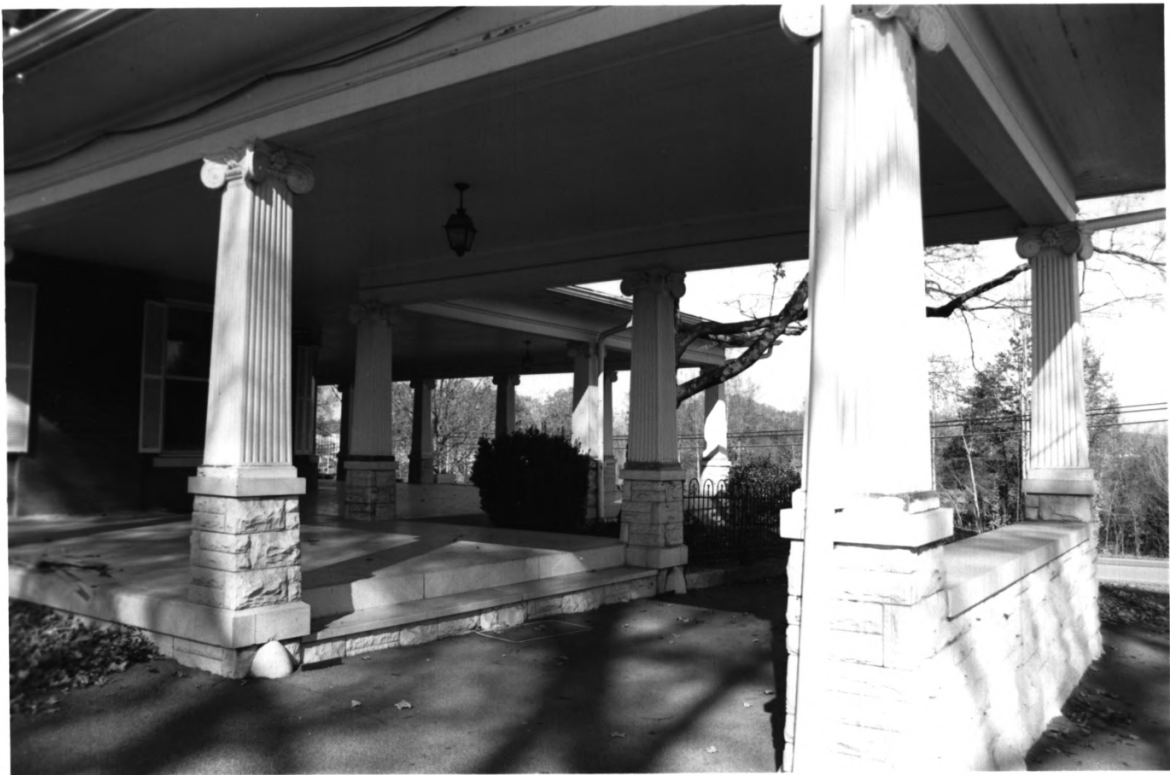
MONDAY HOUSE KNOX COUNTY, TN
