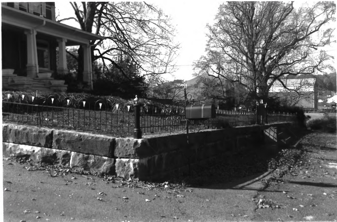
MONDAY HOUSE KNOX COUNTY, TN
