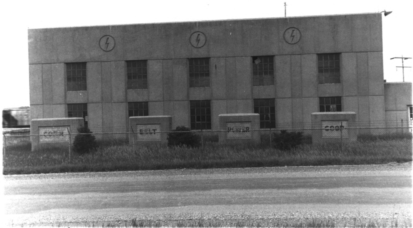
REA PLANT - Franklin Co., Iowa - Item VI, Photo A. Looking north.
