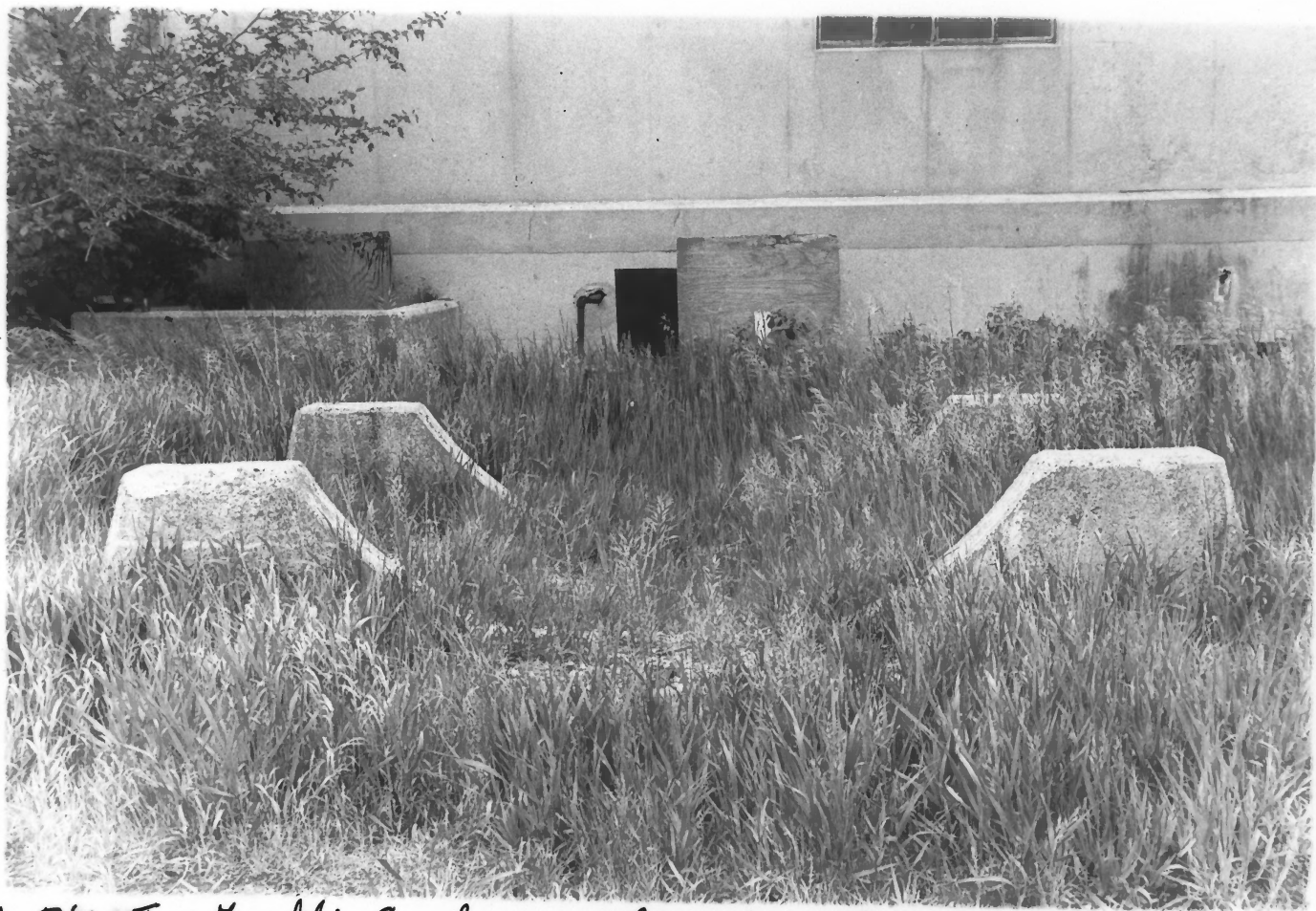
REA PLANT - Franklin Co., Iowa - Item VI Photo C, Fuel tank location.
