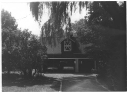
1950 barn/garage at 88 Allendale Road, looking S. neg. file #4-4A.
