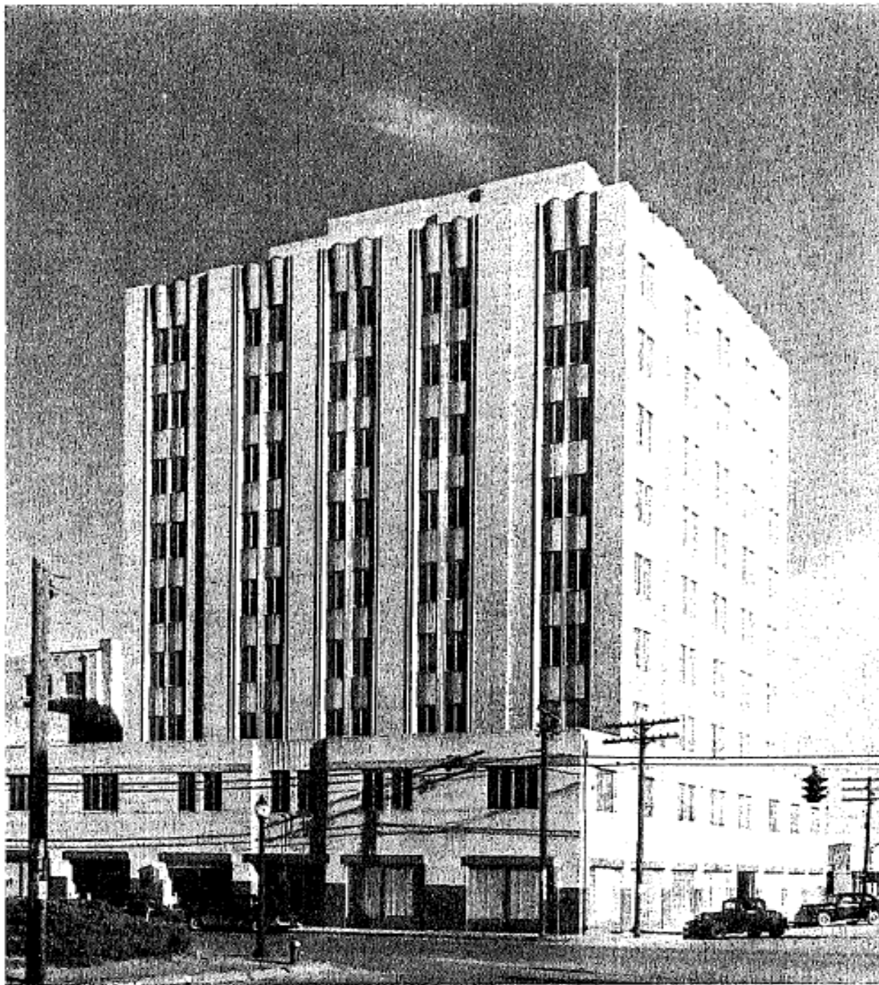
Figure 5 – Midland Tower, early 1950s, from building owner’s files
