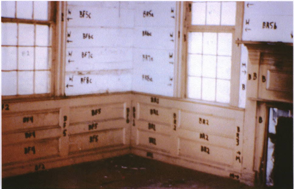
Figure 4. Sample of documentary photograph made prior to the house being moved; note how every piece of wood was numbered for record-keeping and restoration.
