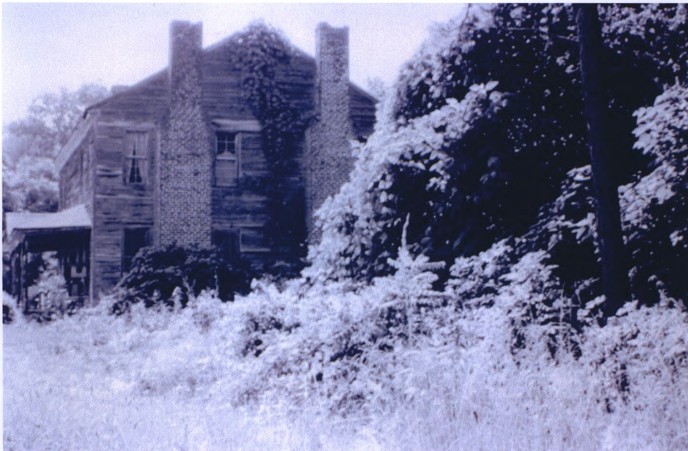
Figure 2. Historic photograph of the Isaac Adair House at its original location prior to being moved for the construction of a new shopping center.
