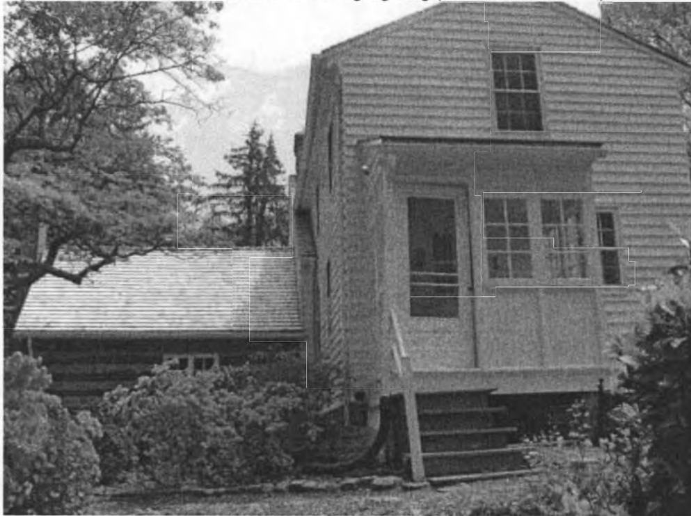
Figure 1.8, South end of west elevation showing original house and 1930s porch (M-NCPPC Collection)
