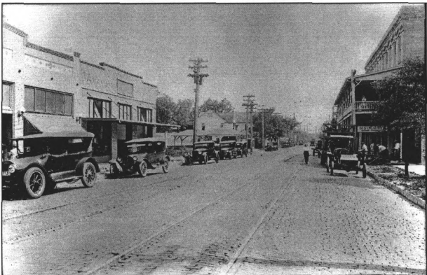
ATTACHMENT 6 , Burgert Brothers Photographers, Building at 1609 North Franklin Street, May 17, 1921, Negative No. 6219.
