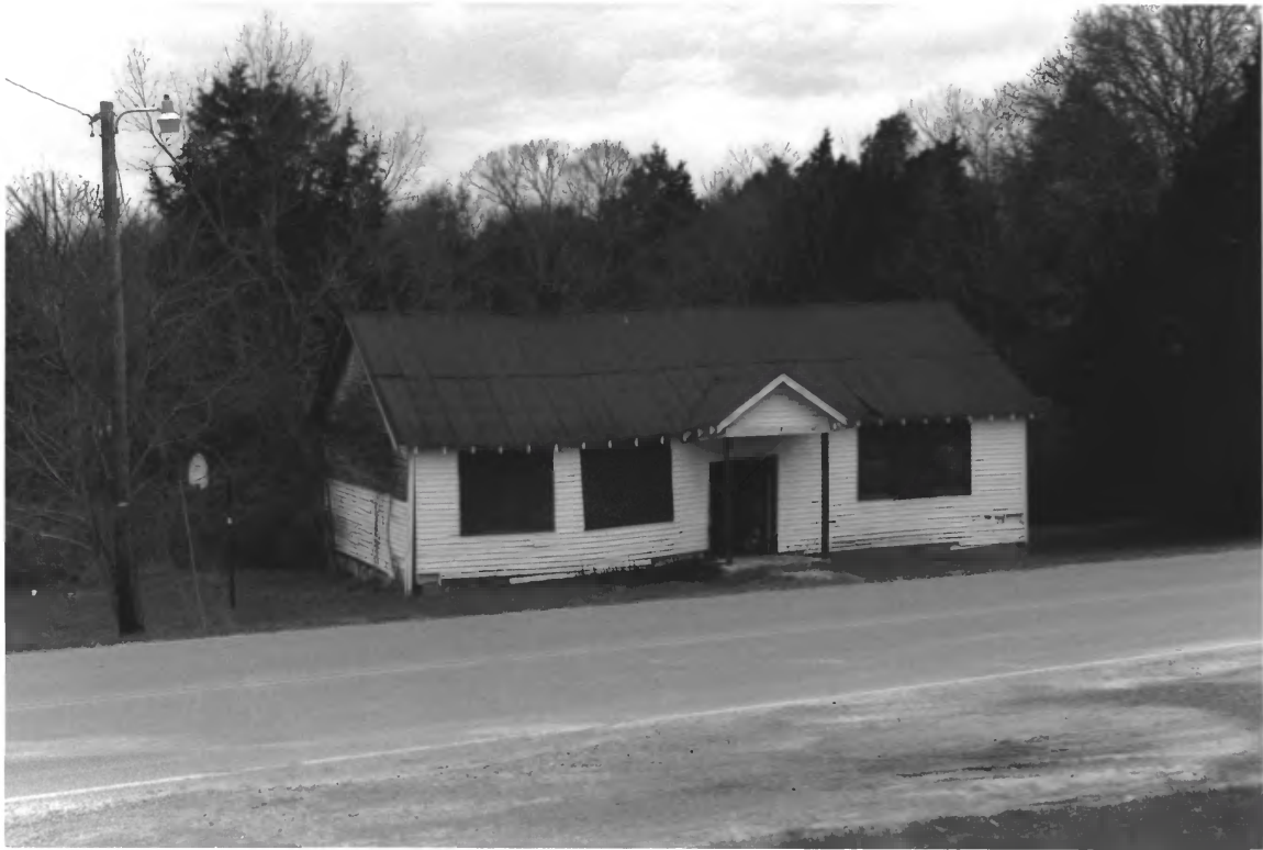
WILLIAMSON CHAPEL CME CHURCH COMPLEX 190F22 WILSON COUNTY TN
