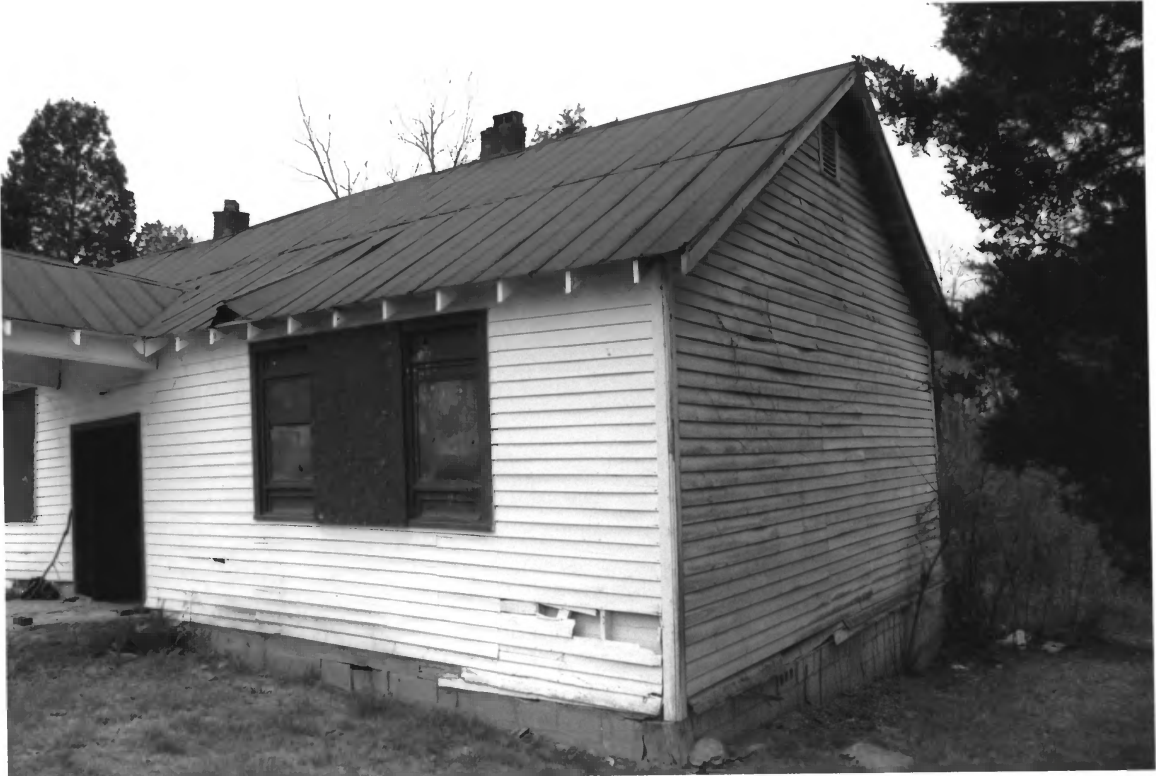
WILLIAMSON CHAPEL CME CHURCH COMPLEX 170F22 WILSON COUNTY TN
