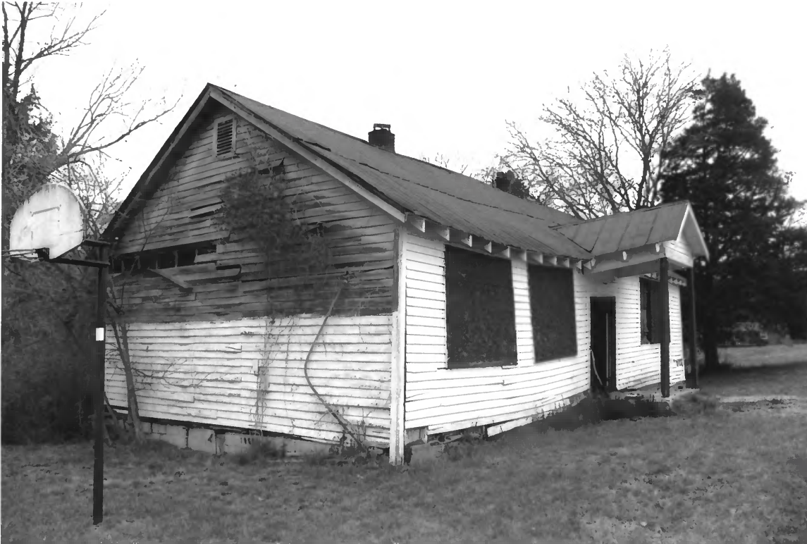
WILLIAMSON CHAPEL CME CHURCH COMPLEX 160F22 WILSON COUNTY TN
