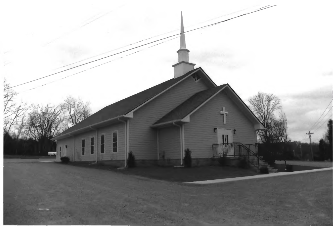
WILLIAMSON CHAPEL CME CHURCH COMPLEX 220F22 WILSON COUNTY TN
