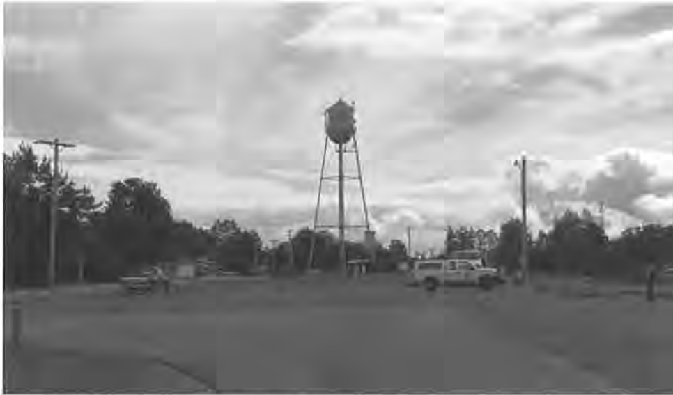
(SOURCE: AKAY Consulting , Floodwood, MN, September 2014)
