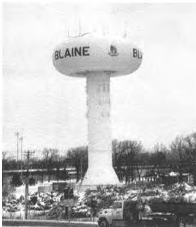
(SOURCE: http://www.mikiemetric.net/USAPics/Water%20Towers/BlaineDonutTower.jpg . Accessed 02/25/2015)
