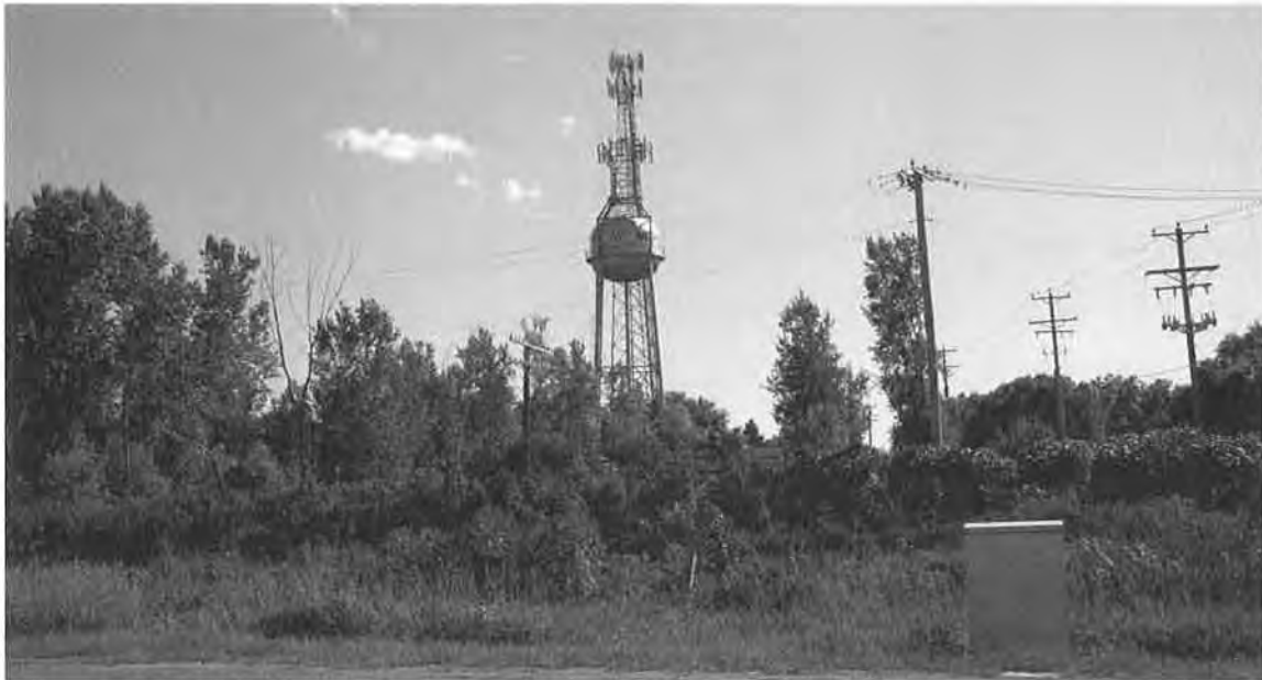
(SOURCE: AKAY Consulting, Medina, MN, September 2014)
