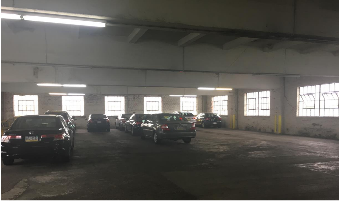
9. Third Floor, view SW
