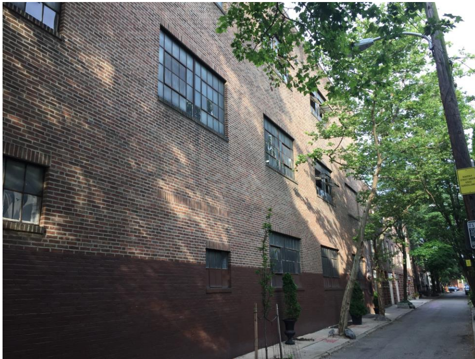
2. North elevation, view SW, from Waverly Street.
