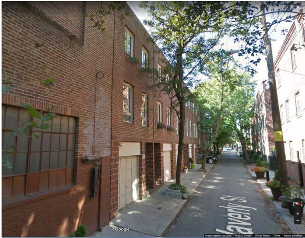
Figure 17: Rear north corner of garage, showing infill rowhomes immediately west of garage's west wall; view facing west along Waverly Street. Note the trend to incorporate garages into new residential construction.
