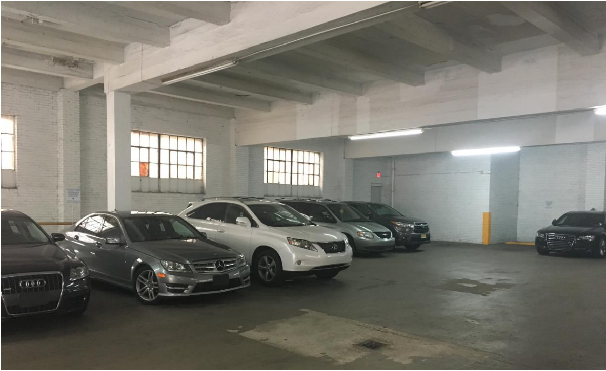
5. First floor, view SW
