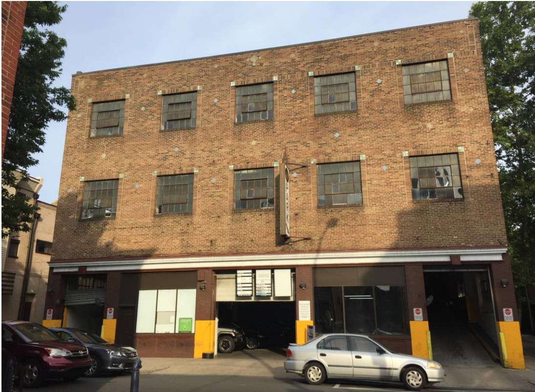
1. East (primary) elevation, showing building entrances.
