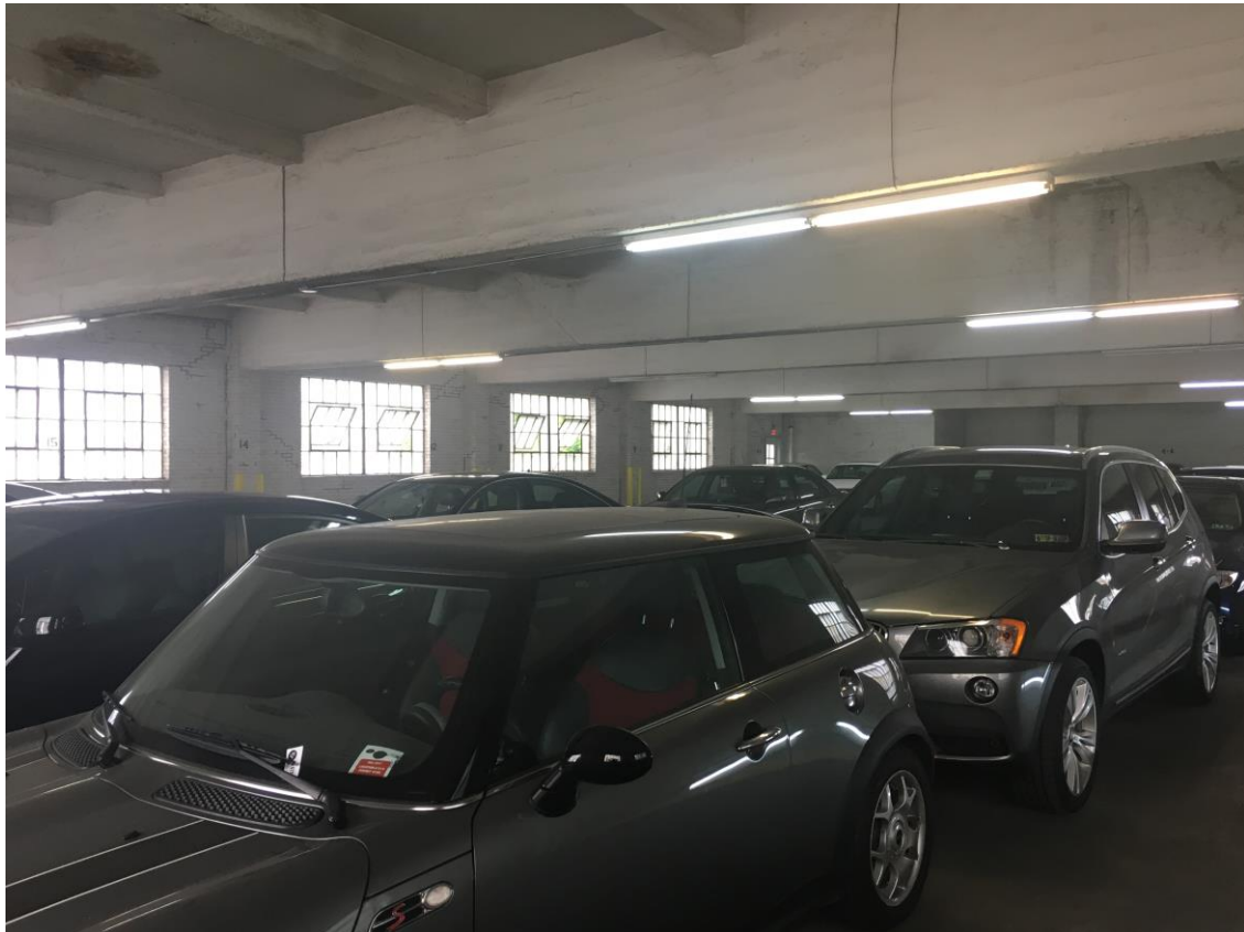
8. Third floor, view SE
