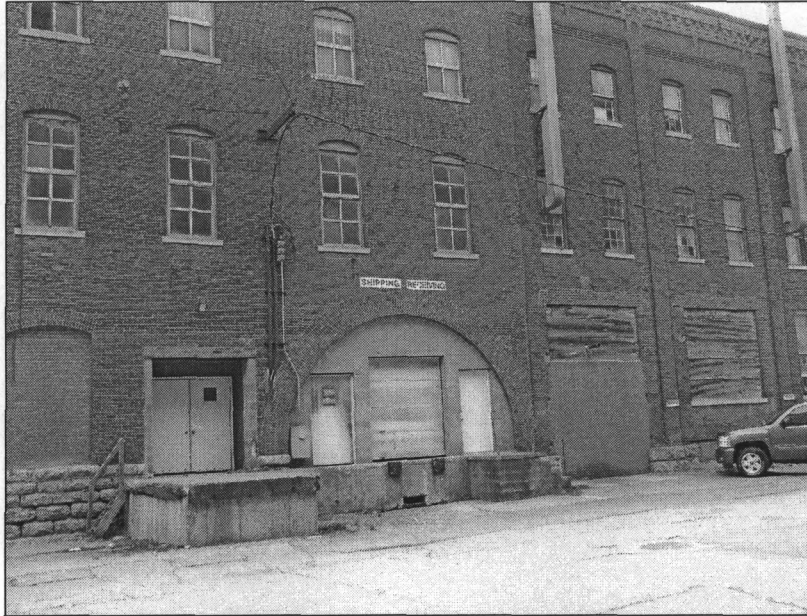
Figure 4: Large semi-circular alleyway door, building #9, north side, view southwest (photo by J. Jacobsen, September 2007)
