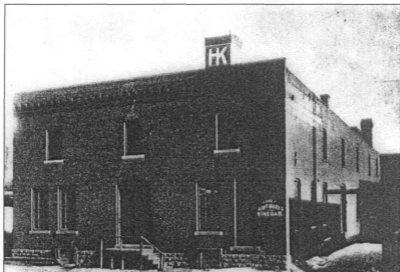
Figure 63: Wicneke-Hohenadel Company, building #15, view northeast (Gardner, 1911).
