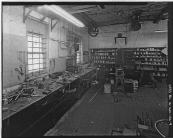
Figure 71: Key City Ironworks (HABS-31-DUBU-13-AK)
