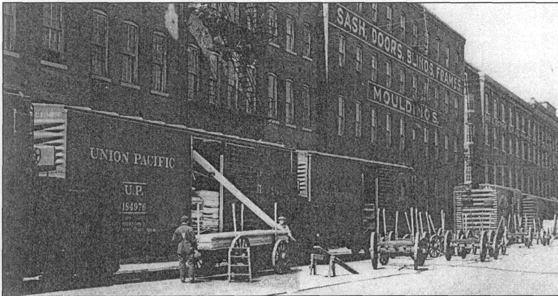
Figure 14: Building #13 is visible to the far right, the block in the foreground is non-extant, view northwest along Jackson Street, from near 7 th Street, April 1940 (Photo by John Vachon, http://memory.loc.gov/ammem/index.html )
