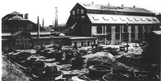
Attachment F – ca. 1900 photo Poole & Hunt Foundry and Machine Works (B-1007) 3500 Clipper Road Baltimore, Maryland Source: Research Center, Baltimore Museum of Industry
