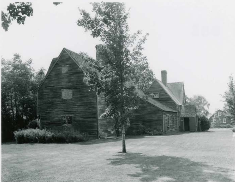
Iron Master's House, 1643 East South End (Left) and West (Rear) Elevation North
