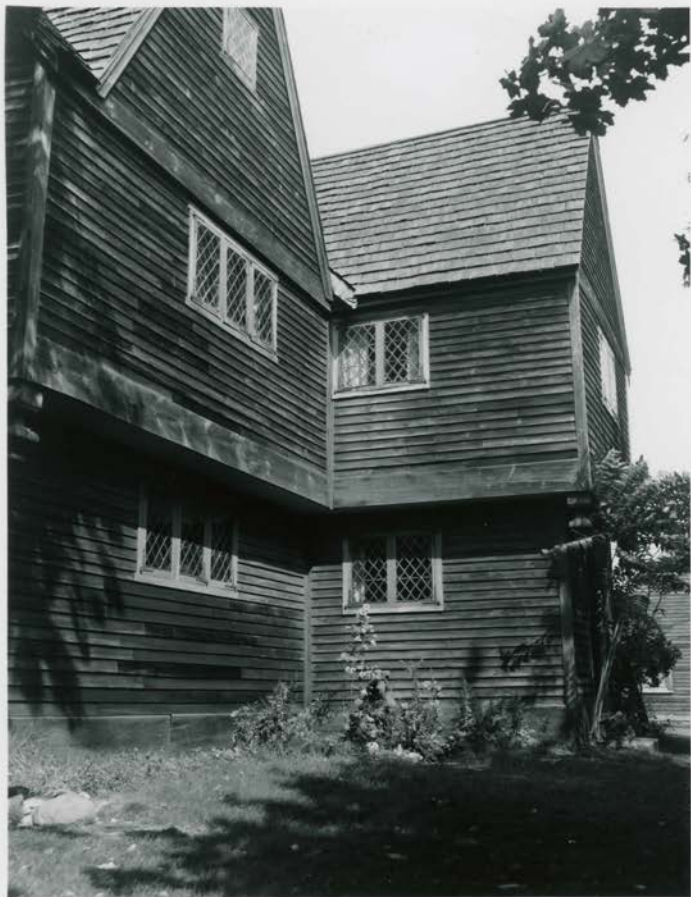
Iron Master's House, 1643 South West (Front) Elevation, Looking South East
