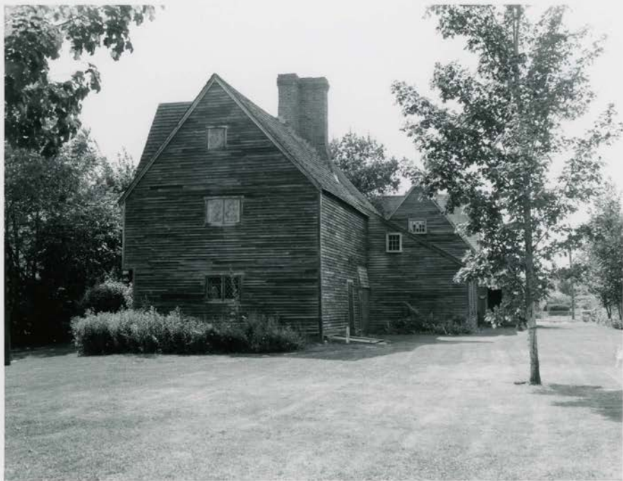
Iron Master's House, 1643 East South End (Left) and East (Rear) Elevation North
