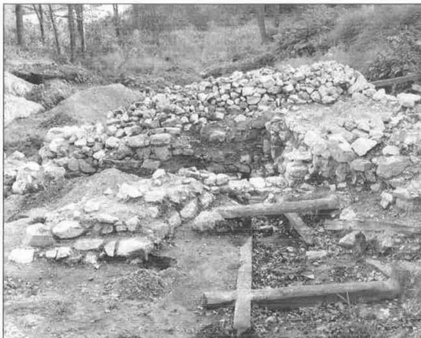
Figure 5. Ca. 1949 photo of excavation of the Blast Furnace bellows base, (source: First Iron Works Association Archives, Saugus Iron Works NHS, Saugus, MA).
