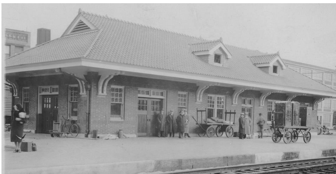
Figure 13b. 1930 Passenger Depot, Main Street (#44), Photo undated
