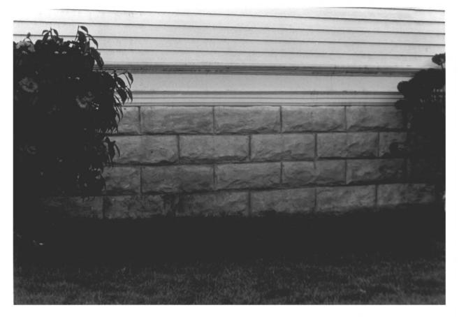
11 of 12 Detail of concrete block foundation simulating rock-faced ashlar. Each unit measures 8x16".
