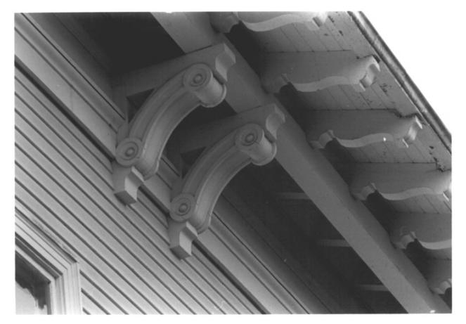
10 of 12 Detail of overhanging eaves carried by outriggers and triangular brackets
