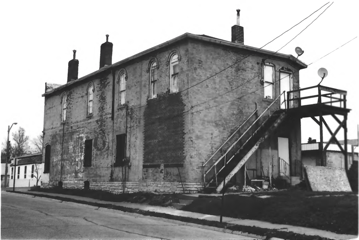
SMITH & WELLER BUILDING HENRY COUNTY, IA #3
