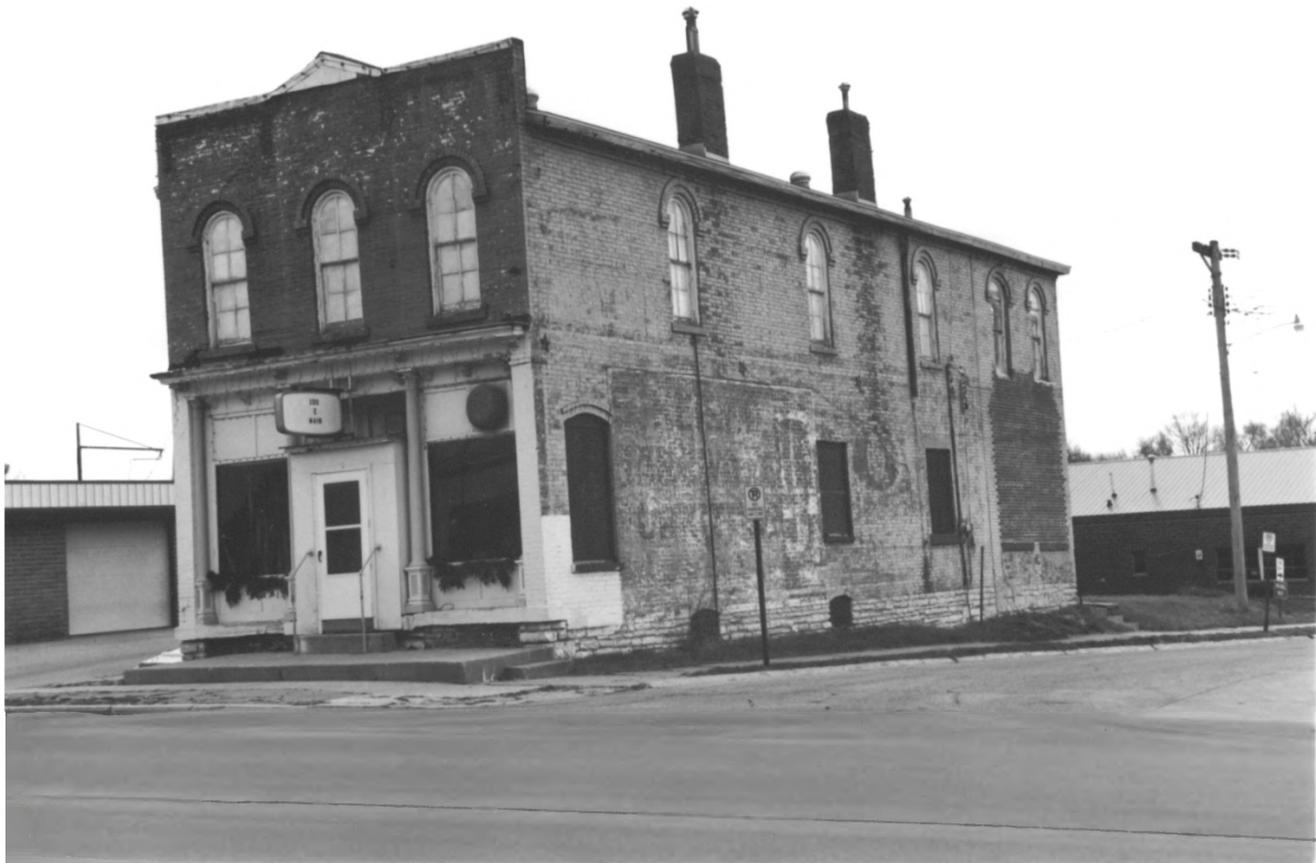
SMITH & WELLER BUILDING HENRY COUNTY, IA #2
