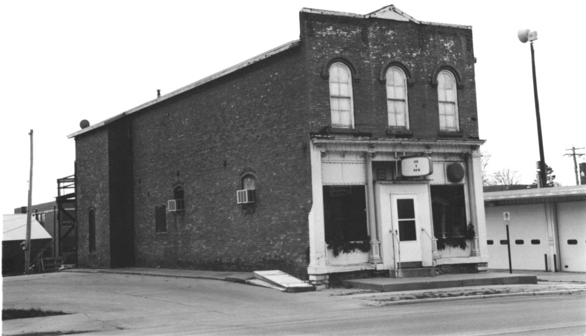
SMITH & WELLER BUILDING HENRY COUNTY, IA # 1
