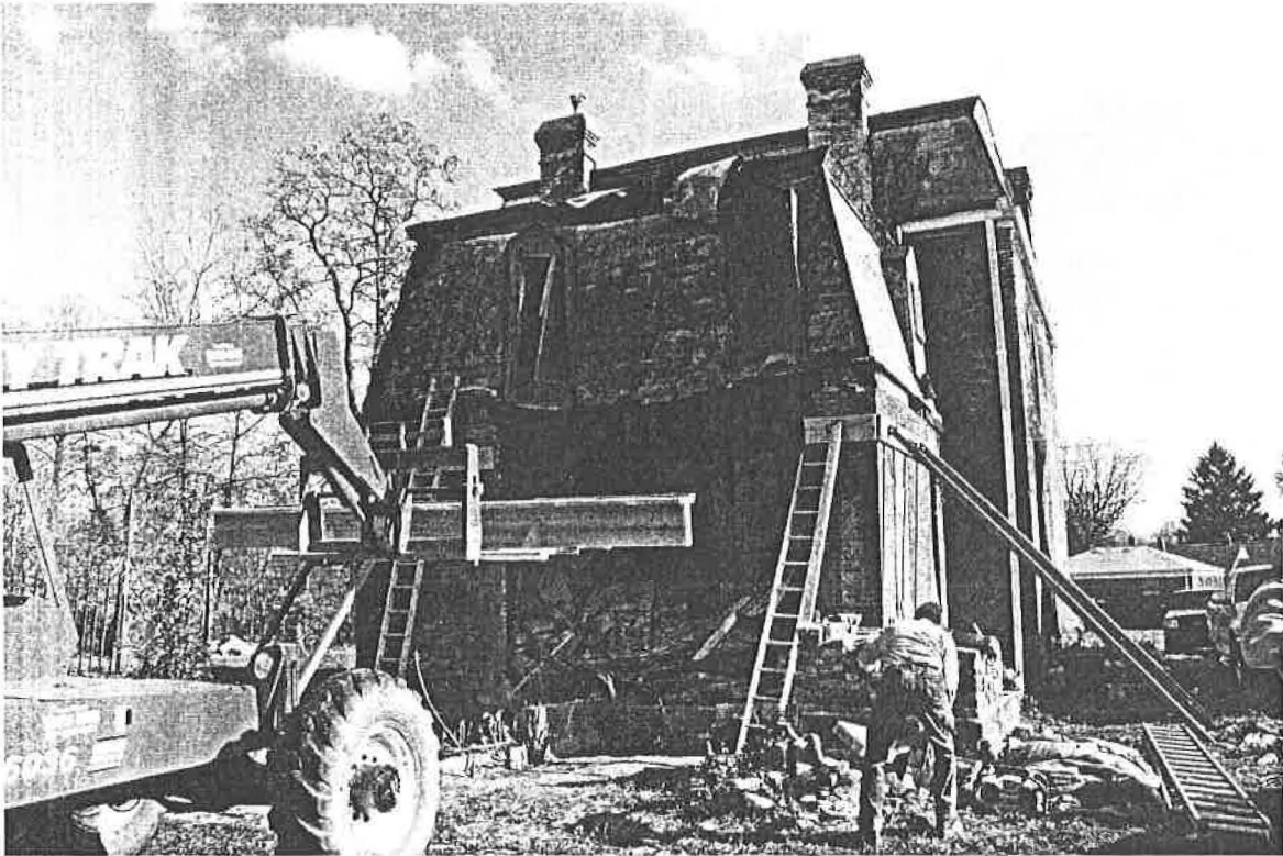
November 10, 2011 installation of support beam
