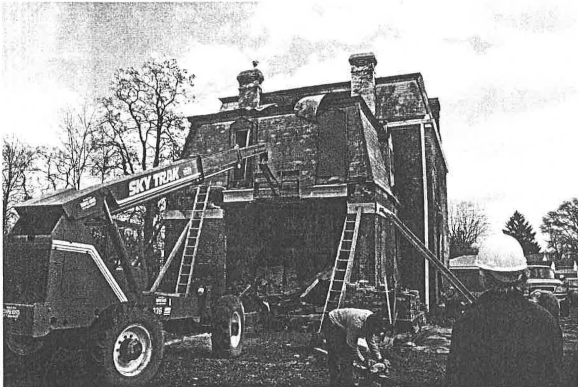
November 10, 2011 installation of support beam
