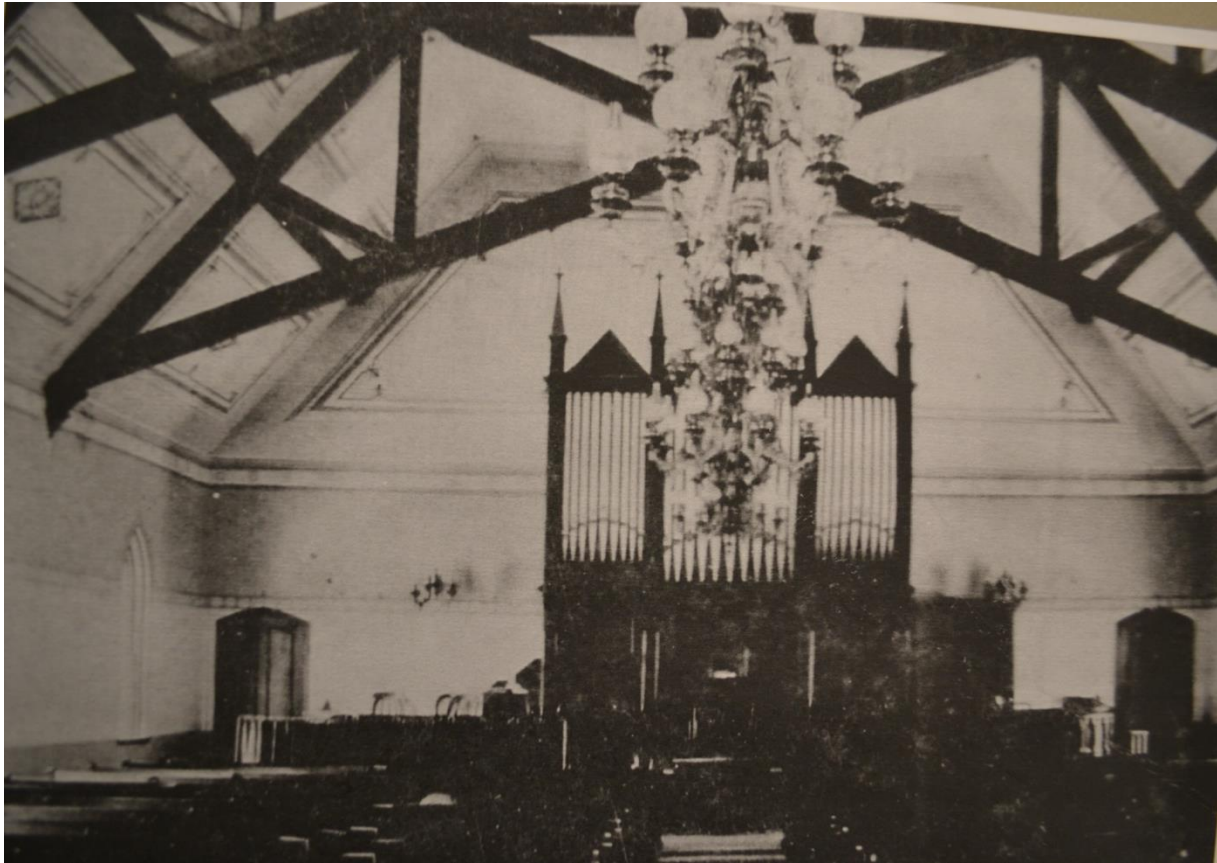
The First Congregational Church, Farmington before the c.1900 addition of pressed tin on the ceiling. The original light fixtures, wall & ceiling stenciling as well as the display pipes and upper portion of the organ case are visible.
