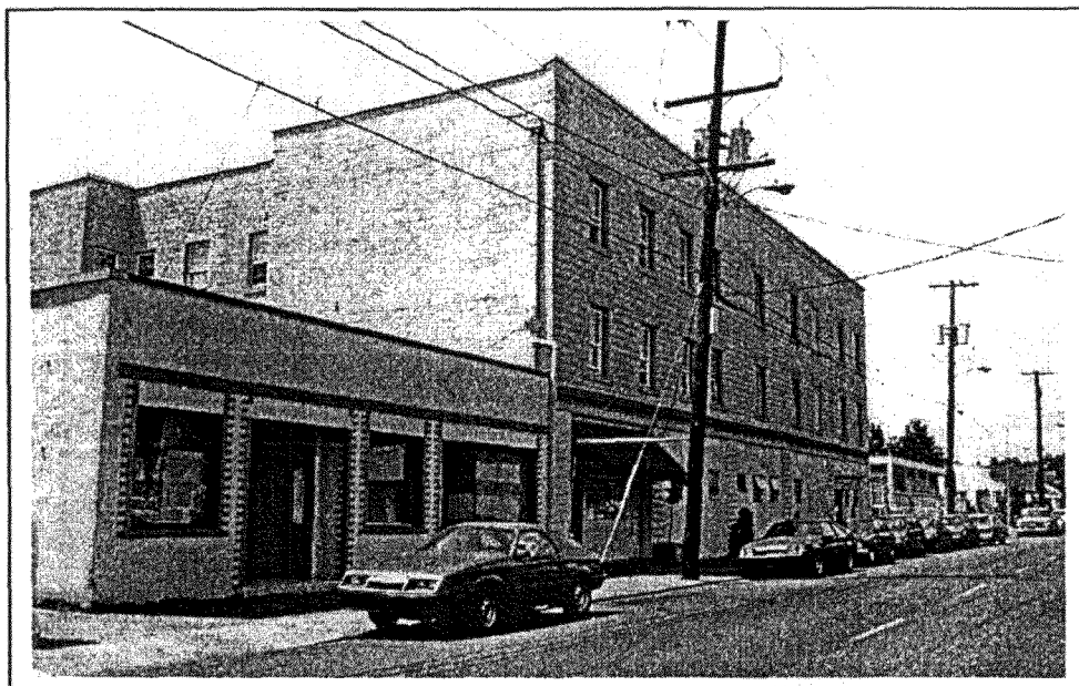
Looking southwest at 2026 N. Kilpatrick Street (Inv. # 26, at left) and 2044 N. Kilpatrick Street (Inv. #27).
