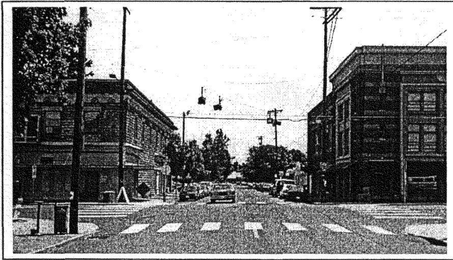
Looking east from N. Kilpatrick Street at 8202-8208 N. Denver Avenue (Inv. #22, at left) and 8130-8134 N. Denver Avenue (Inv. #19).
