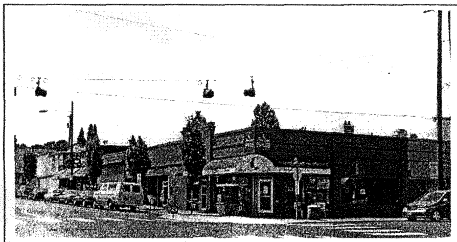
Looking southwest at 8131-8139 N. Denver Avenue (Inv. #8).
