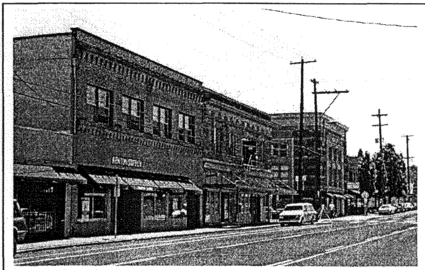
Looking southeast at 8212-8216 N. Denver Avenue (Inv. #23, at left); 8202-8208 N. Denver Avenue (Inv. #22, at center); and 8130-8134 N. Denver Avenue (Inv. #19, at right).
